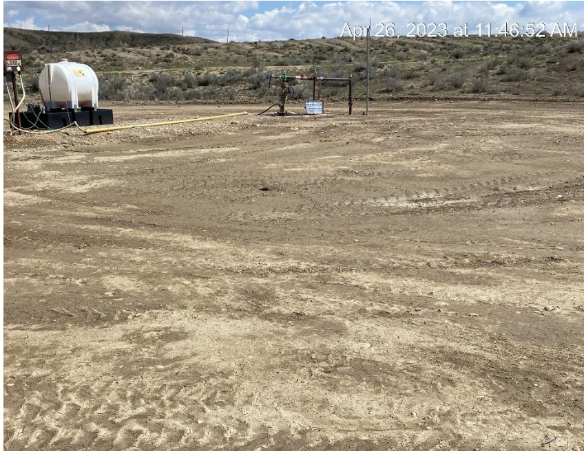
Southwest corner of location
