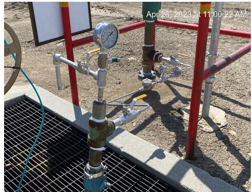
Surface casing hooked into flowline
