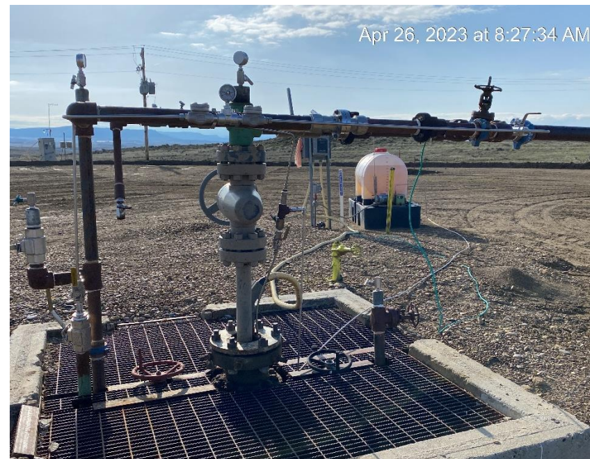
Surface casing hooked into flowline
