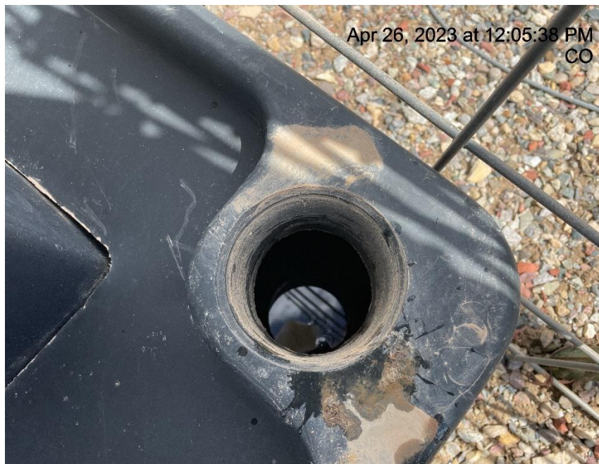
Photo # 6418 Chemical containment is approximately 3/4 full/Failure to maintain chemical BMP
