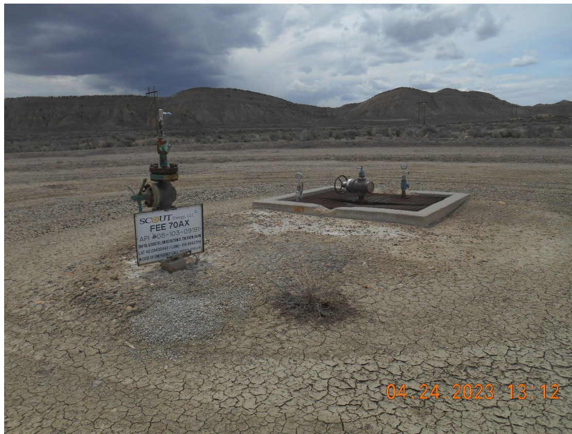
Injection wellhead. Temporarily Abandoned
