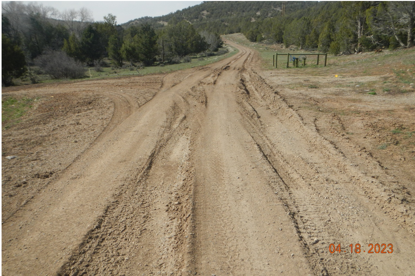
Photo 1. Facing northwest along the access road. There is vehicle rutting and tracking along the road that needs to be repaired and stabilized.
