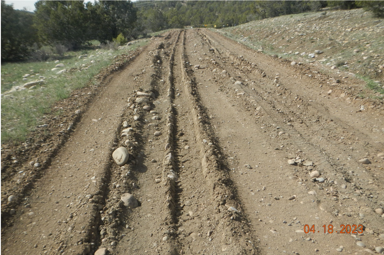
Photo 1. Facing northwest along the access road. There is vehicle rutting and tracking along the road that needs to be repaired and stabilized. Gate was locked and couldn't go any further.
