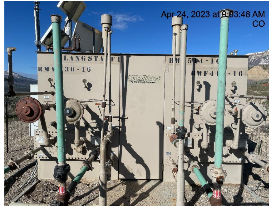
Photo # 6067 Meter calibration info not conspicuously posted
