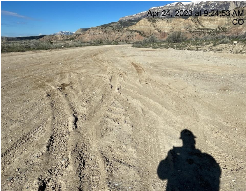
Photo # 6108 Lack of stabilization/Compaction on location
