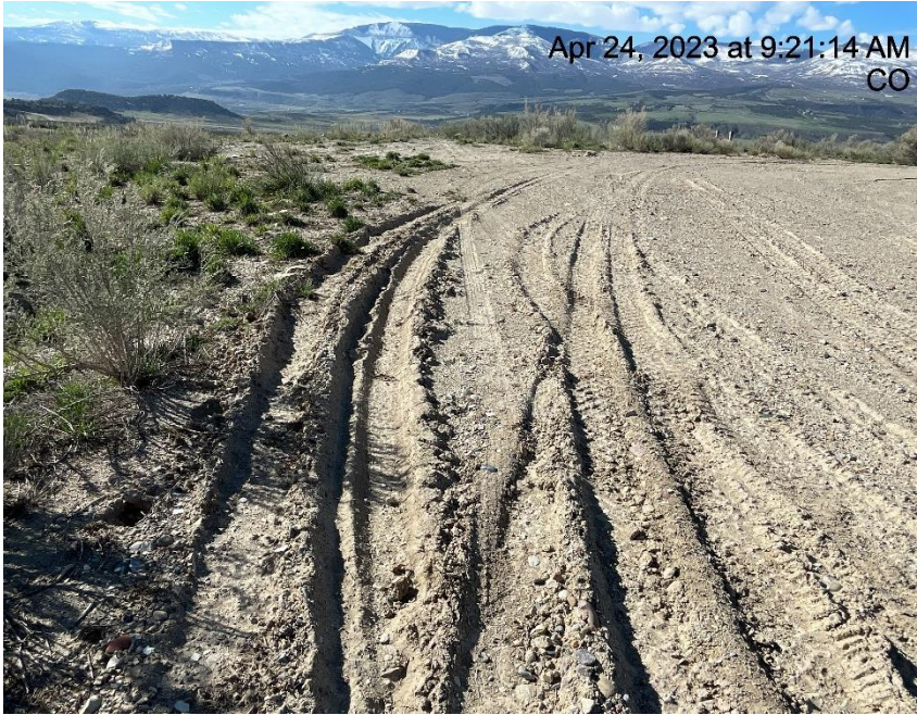
Photo # 6098 Lack of stabilization/Compaction on location
