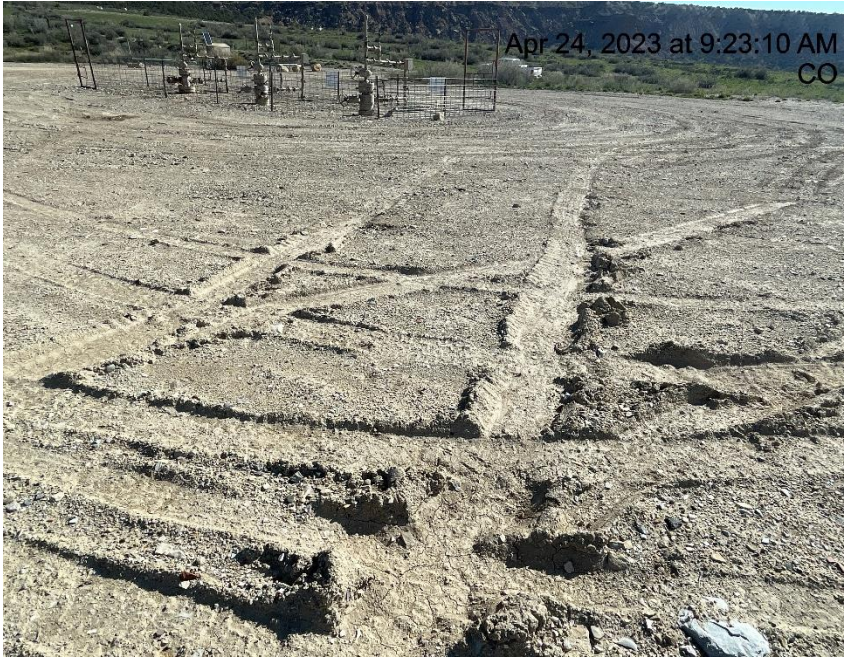
Photo # 6103 Lack of stabilization/Compaction on location
