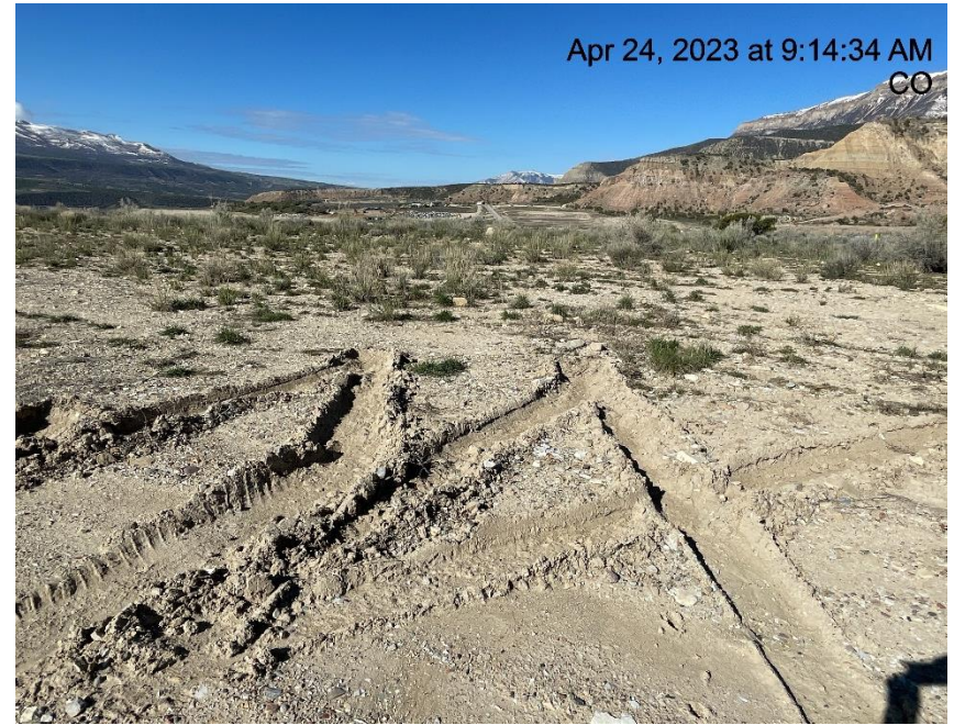
Photo # 6081 Failure to minimize surface disturbance
