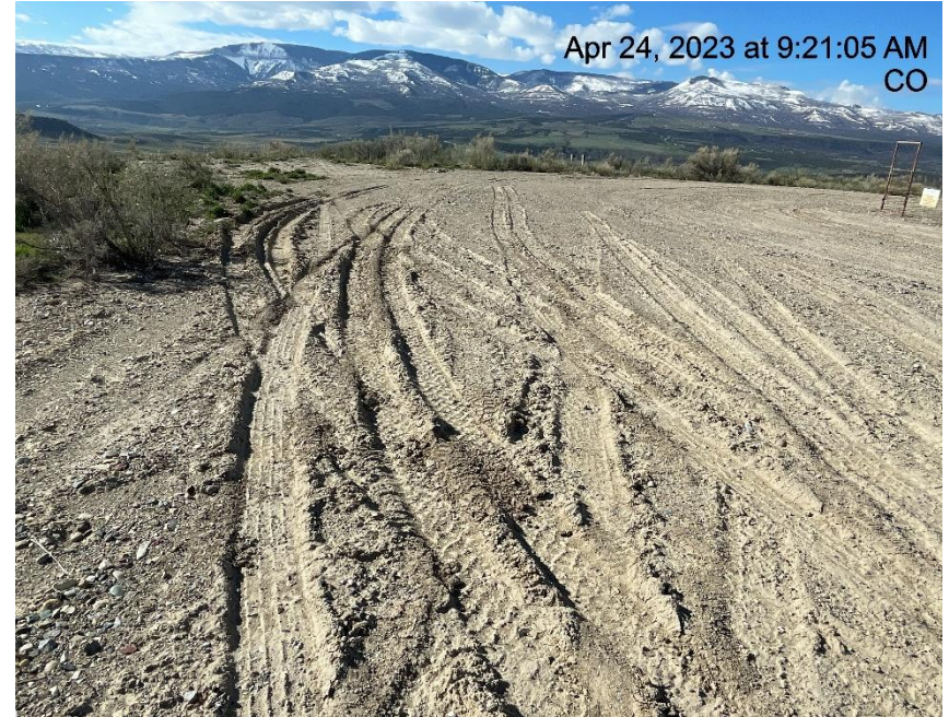
Photo # 6097 Lack of stabilization/Compaction on location
