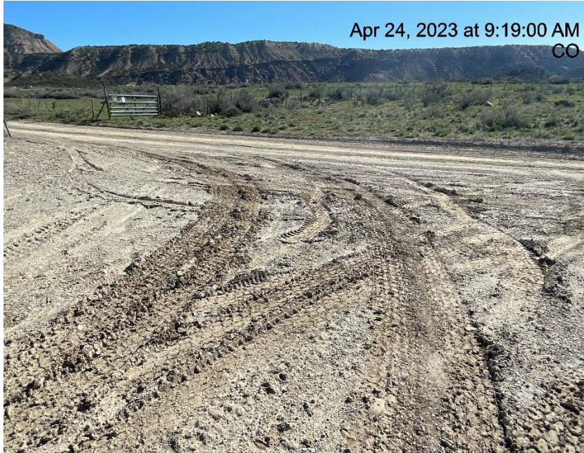
Photo # 6094 Lack of stabilization/Compaction/Insufficient tracking BMP's
