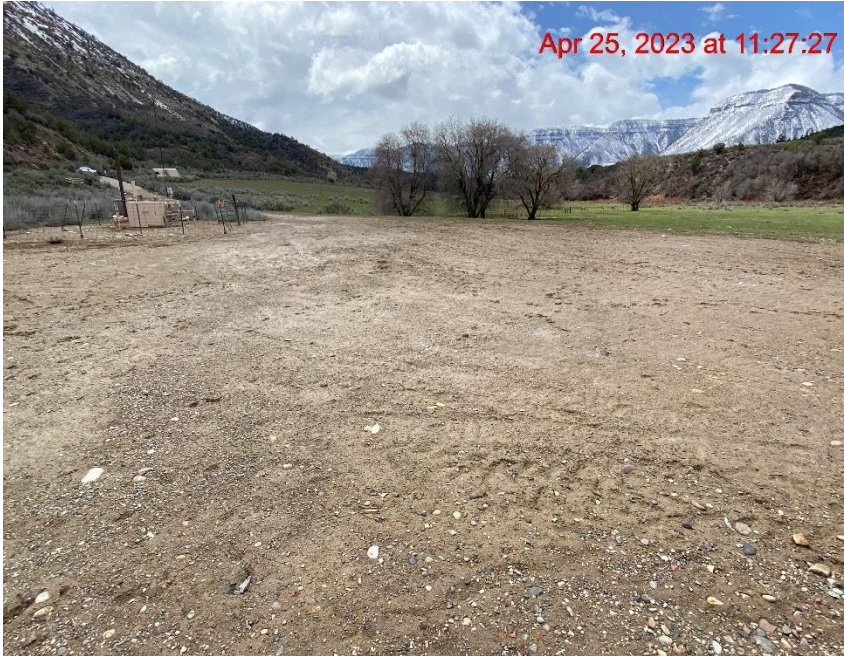
Location Lacks Stabilization – Photo #02554
