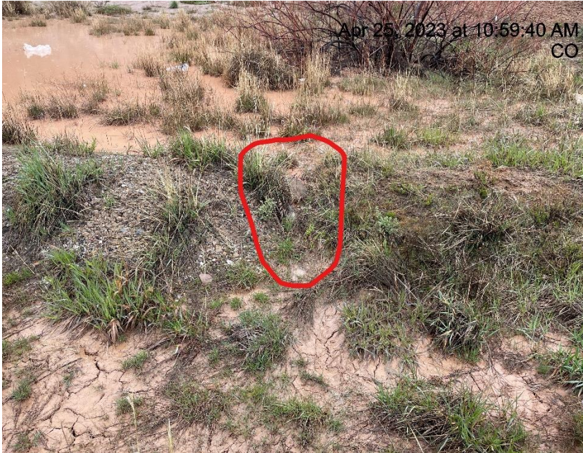
Photo # 6353 Berm needs maintenance/erosion & transport of sediment (E/NE area of berm)
