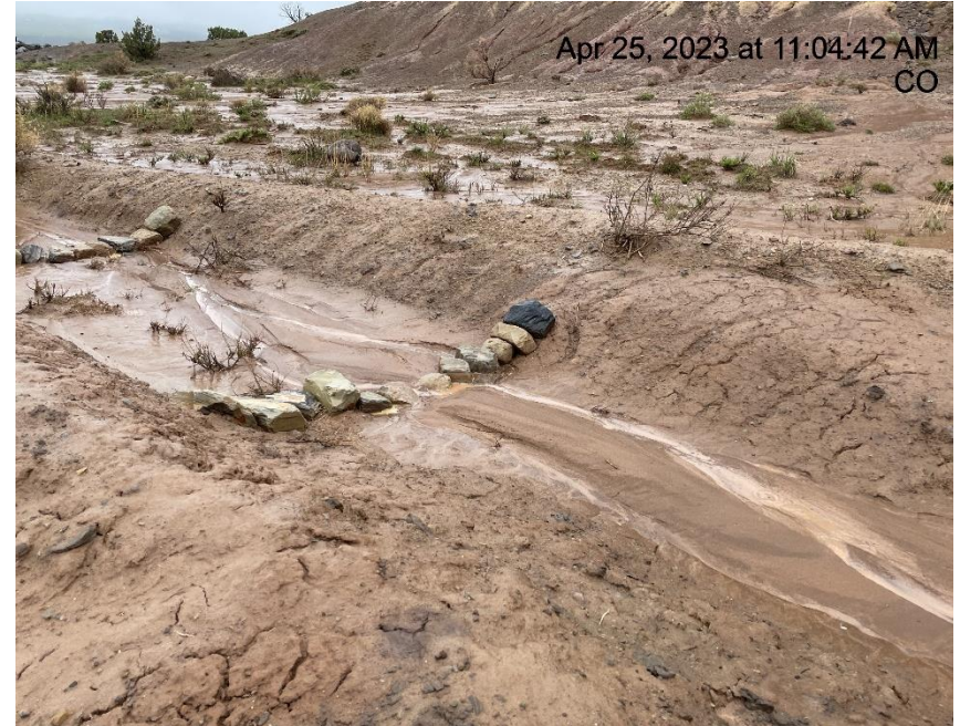
Photo # 6368 Check dams need maintenance
