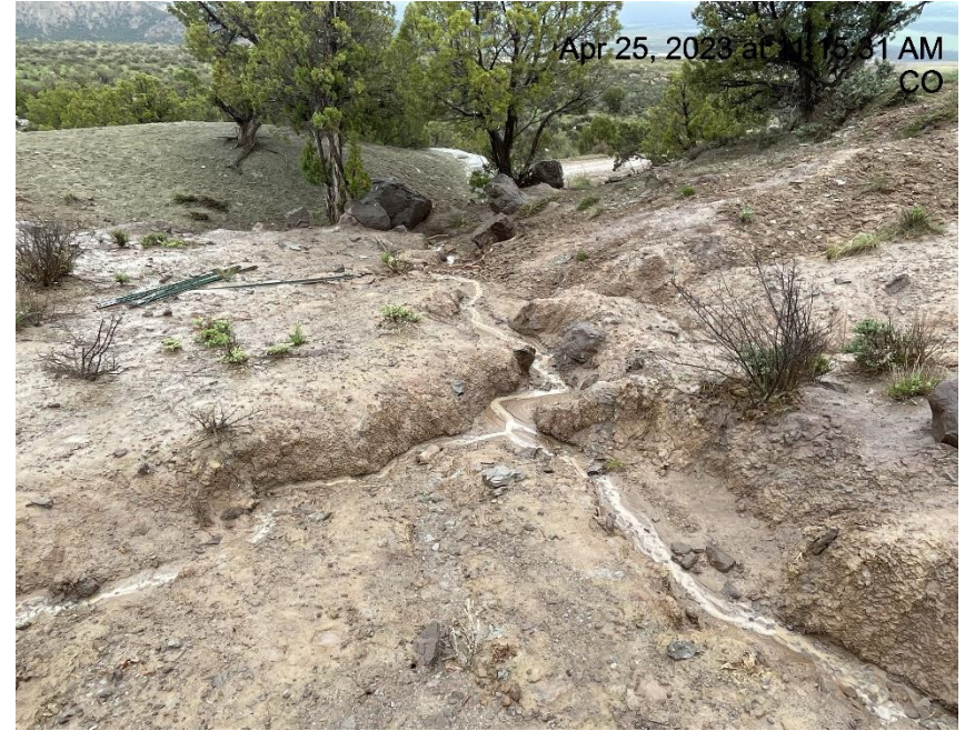
Photo # 6391 Erosion & transport of sediment on slope just off location (S/SW area)
