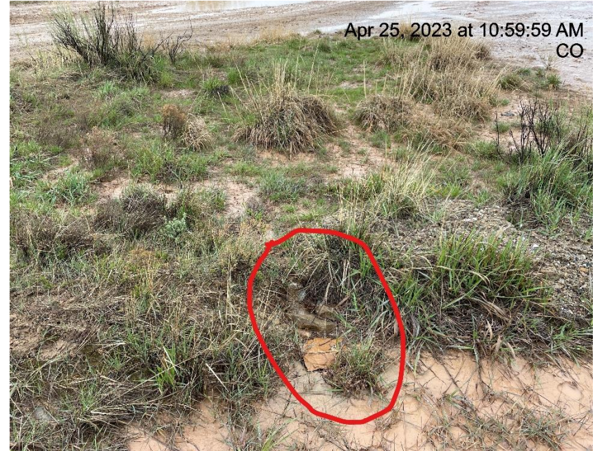
Photo # 6354 Berm needs maintenance/erosion & transport of sediment (E/NE area of berm)
