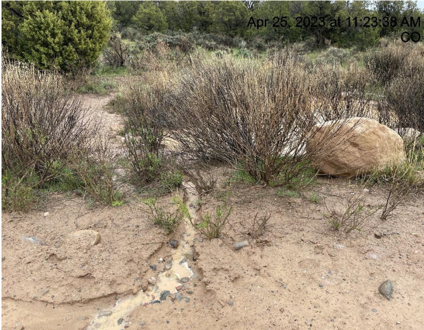
Photo # 6399 Erosion & transport of sediment on edge of location (S/SE area of location)
