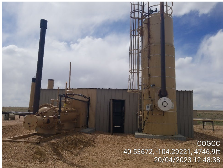
Photo 7 – Separator and Heater Treater
