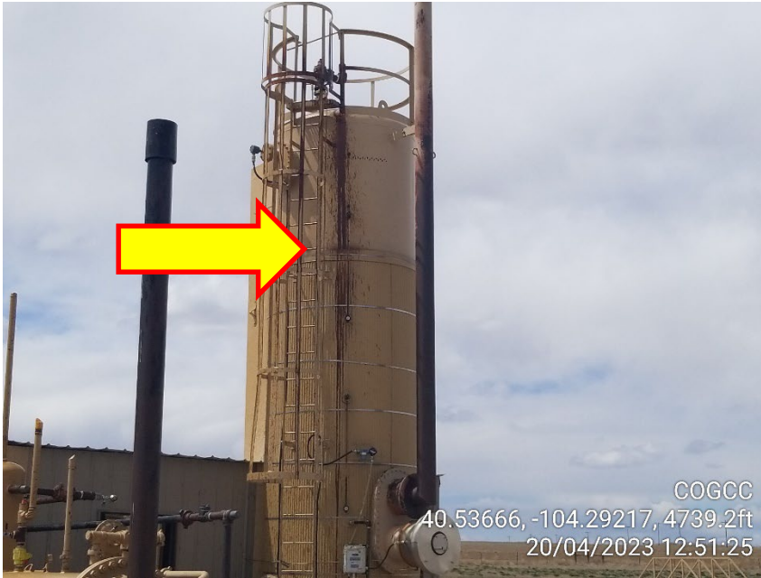
Photo 17 – Unmarked Riser at Gas Meters
