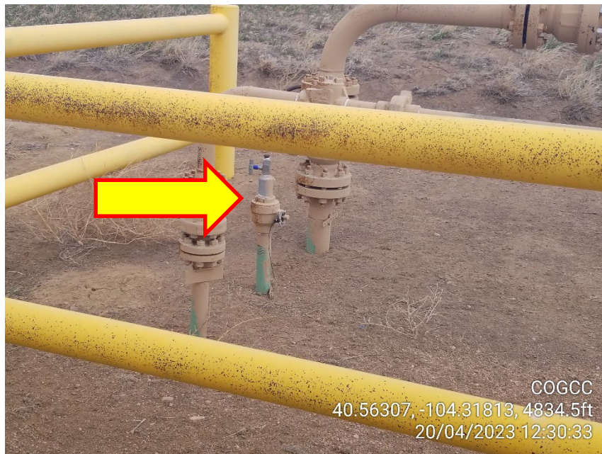
Photo 17 – Unmarked Riser at Gas Meters
