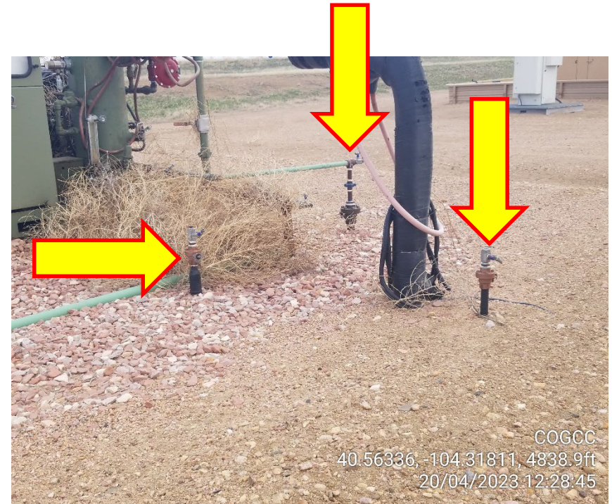
Photo 12 – Unmarked Risers
