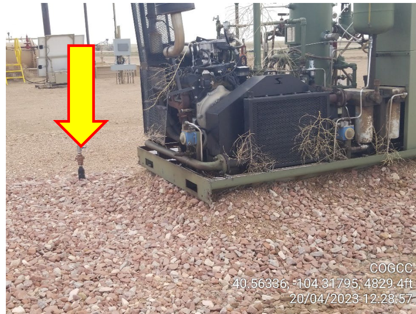
Photo 14 – Unmarked Risers
