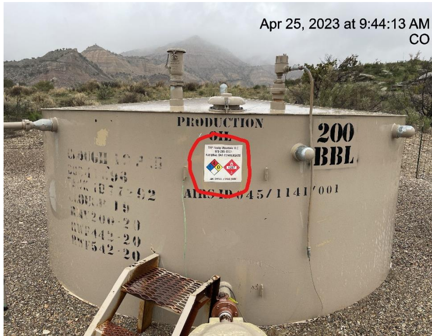
Photo # 6243 Tank label inaccurate/incorrect information
