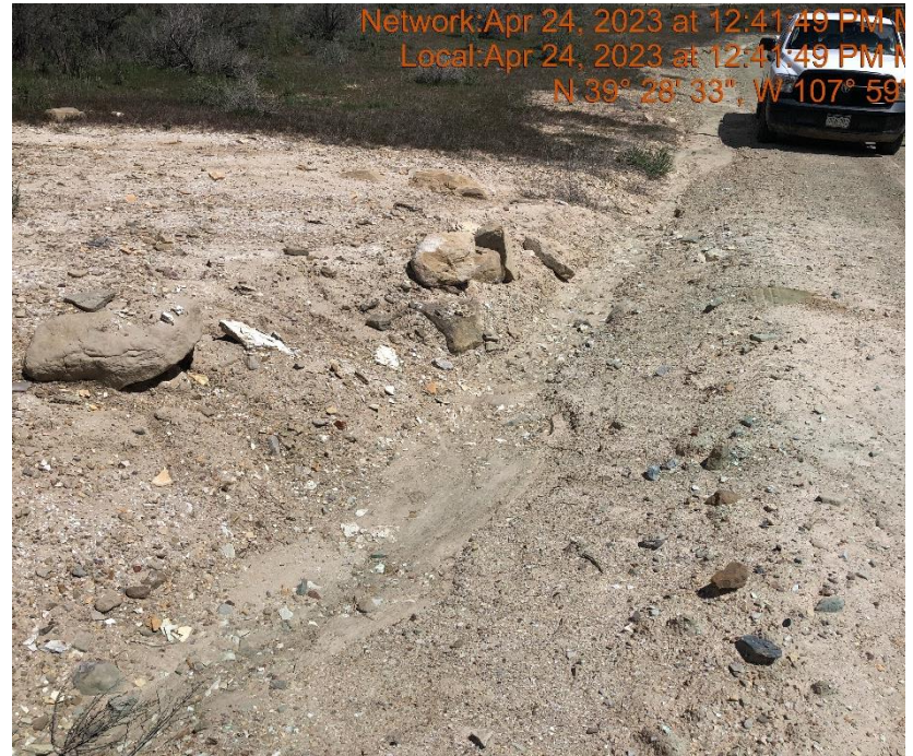
Photo #9717 Insufficient velocity BMP's.
