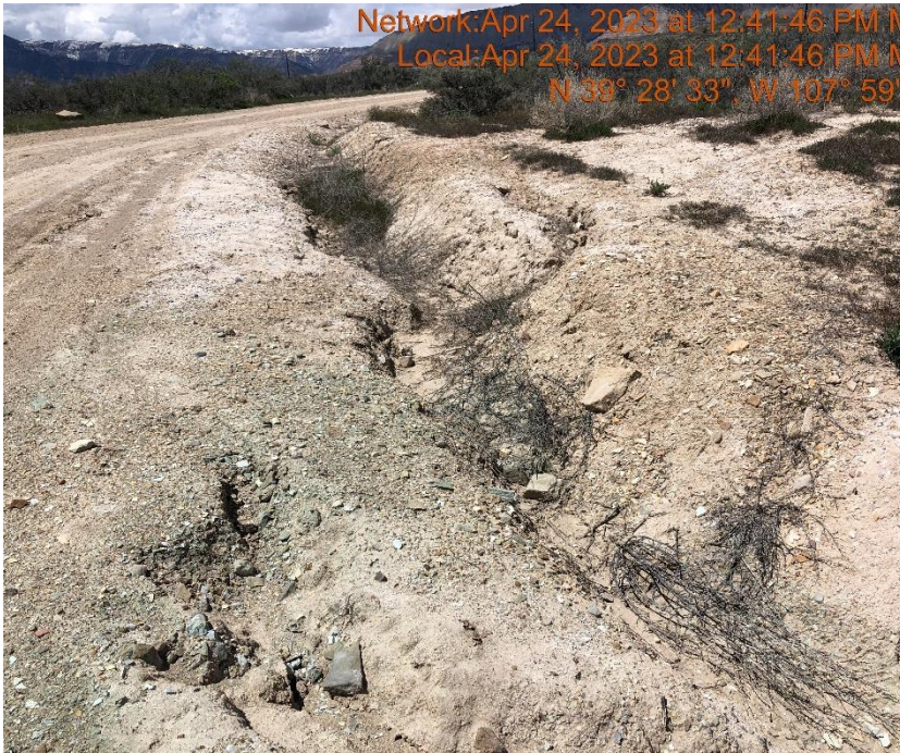
Photo #9716 Insufficient velocity BMP's.
