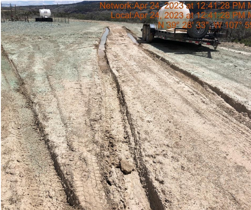
Photo #9715 Location lacks stabilization.
