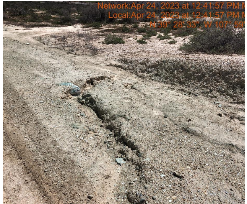
Photo #9718 Rill erosion occurring on location.
