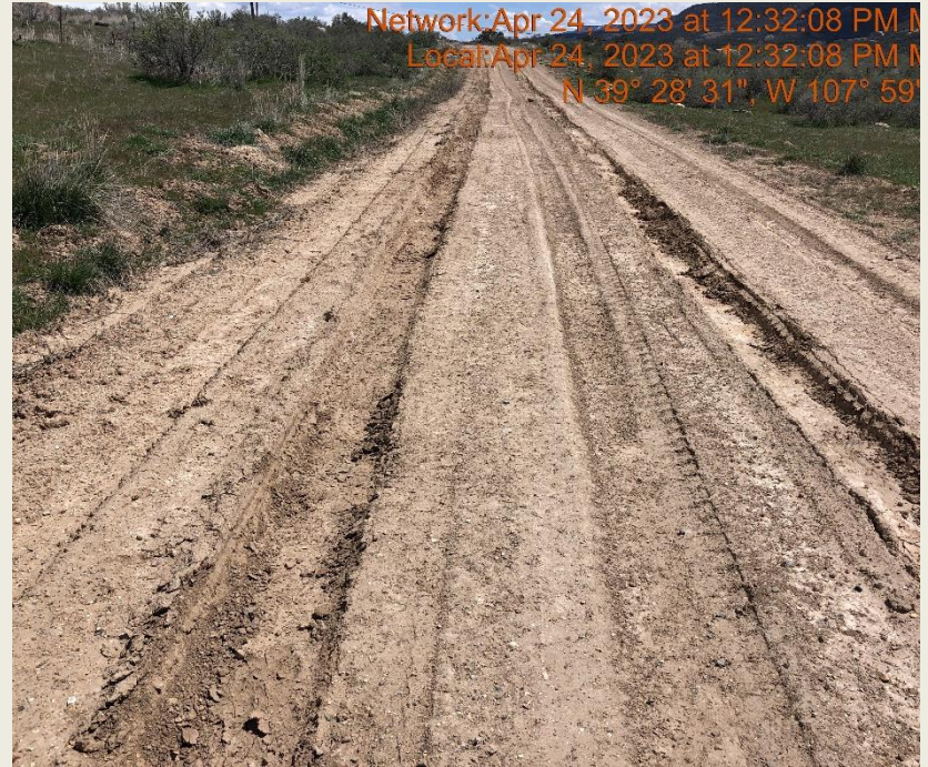
Photo #9707 Access road lacks stabilization.
