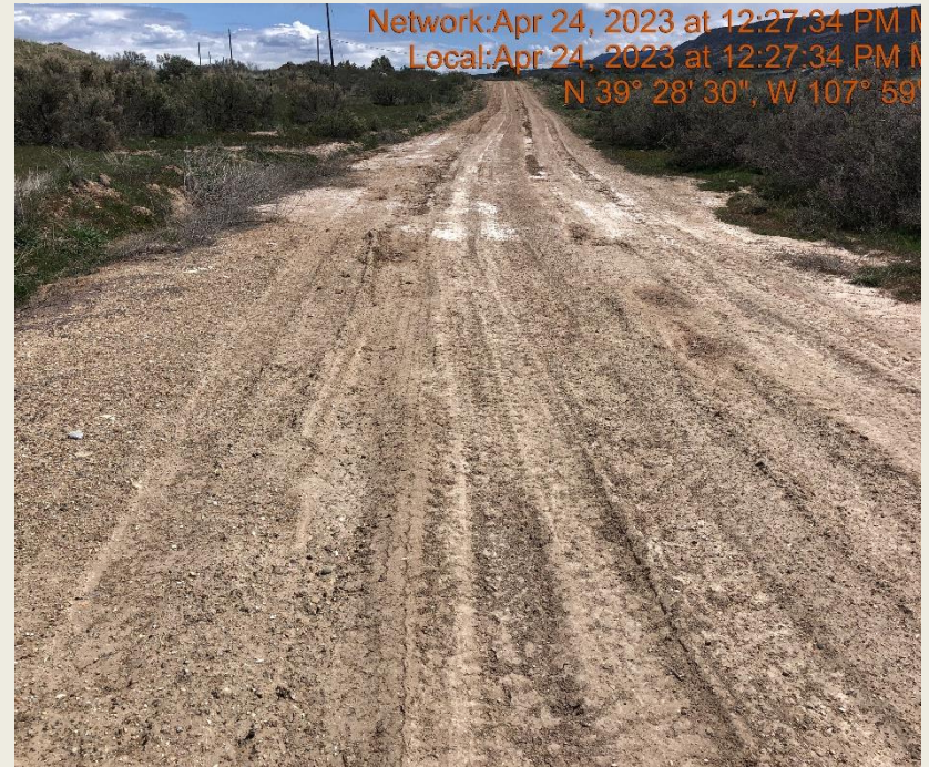
Photo #9702 Access road lacks stabilization.
