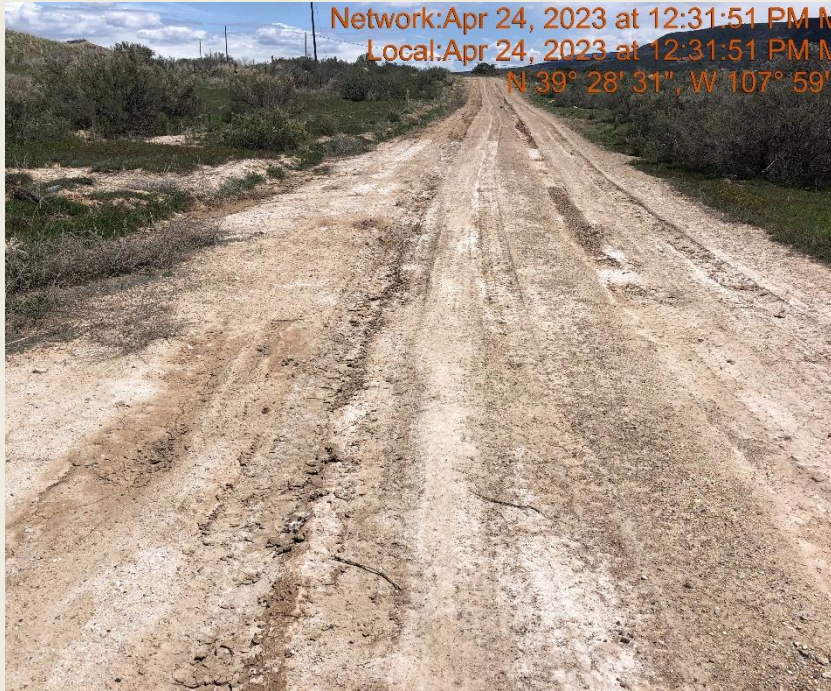
Photo #9706 Access road lacks stabilization.
