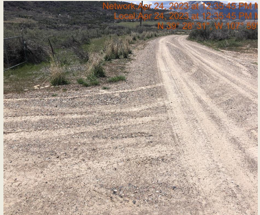
Photo #9709 Insufficient tracking BMP to minimize the transport of sediment.
