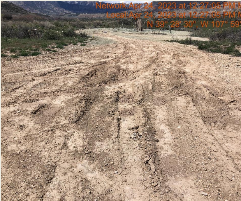
Photo #9700 Access road lacks stabilization.
