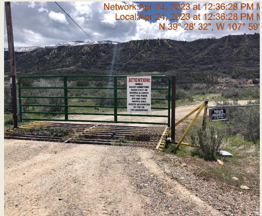
Photo #9711 Insufficient tracking BMP to minimize the transport of sediment.
