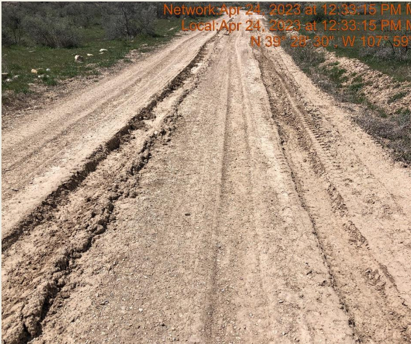
Photo #9708 Access road lacks stabilization.
