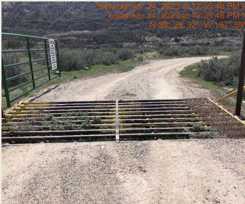
Photo #9710 Insufficient tracking BMP to minimize the transport of sediment.
