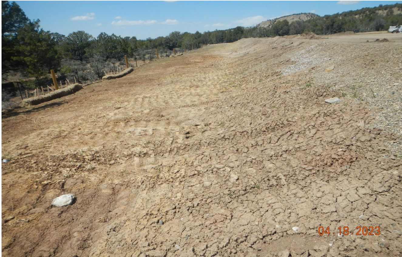
Photo 7. South side of the location facing west along the fill slope. It appears track was redone perpendicular to the slope and soils were seeded and hydromulched.
