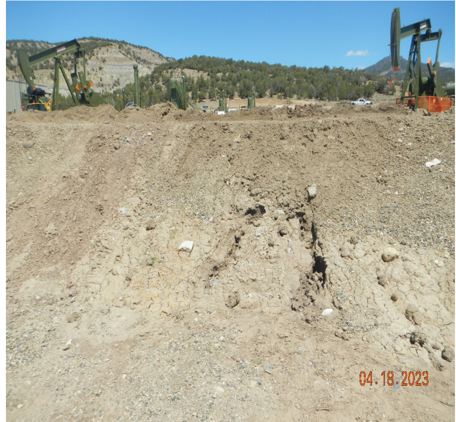
Photo 9. There was erosion that occurred off the midway of the pad. The erosion was graded back in but should be better stabilized to prevent erosion in this area.
