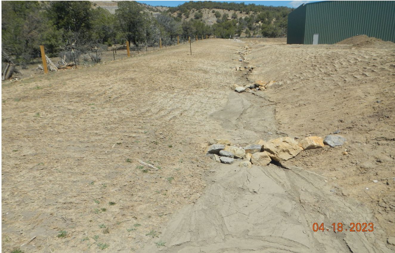
Photo 10. Southwest corner of the pad facing north. The rock check dams are slowing down stormwater flow but need maintenance to prevent washing out underneath or around the check dams.
