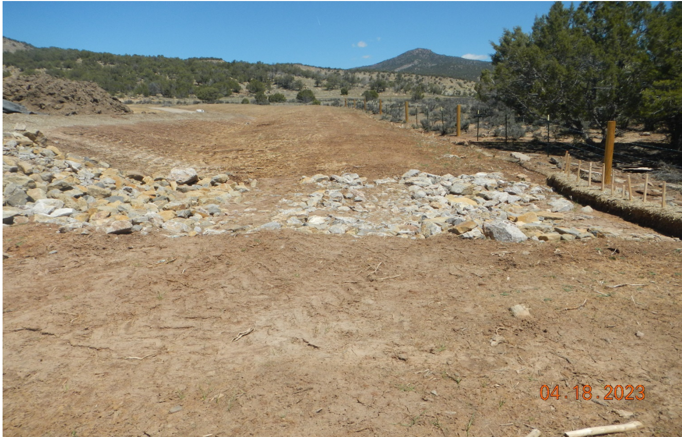
Photo 6. Southeast corner of the location facing north. There has been additional BMP's installed at the southeast corner of the location which is in close proximity to the ephemeral drainage.
