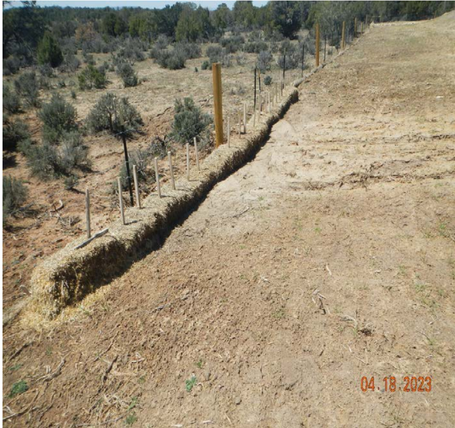
Photo 8. There were straw bales installed at about midway of the pad which have held back sediment. The sediment will need to be cleaned out so it won't overtop the bales.
