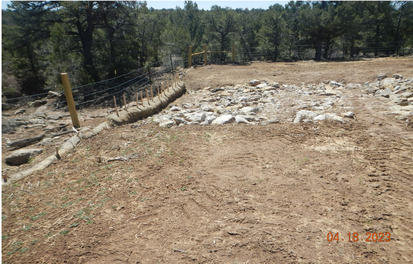
Photo 5. There has been additional BMP's installed at the southeast corner of the location which is in close proximaty to the ephemeral drainage.
