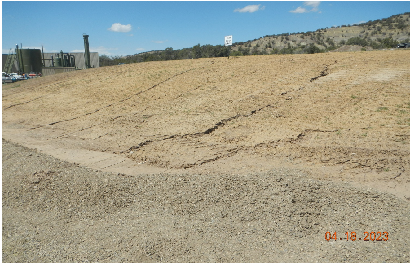
Photo 14. There are some rills beginning to occur along the cut slope. Additional BMP's need to be installed to prevent further erosion.
