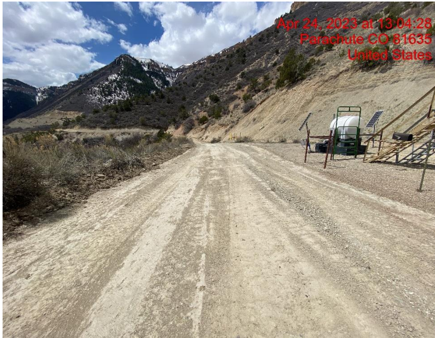
Inadequate Vehicle Tracking BMPs at Location Entrance – Photo #02481
