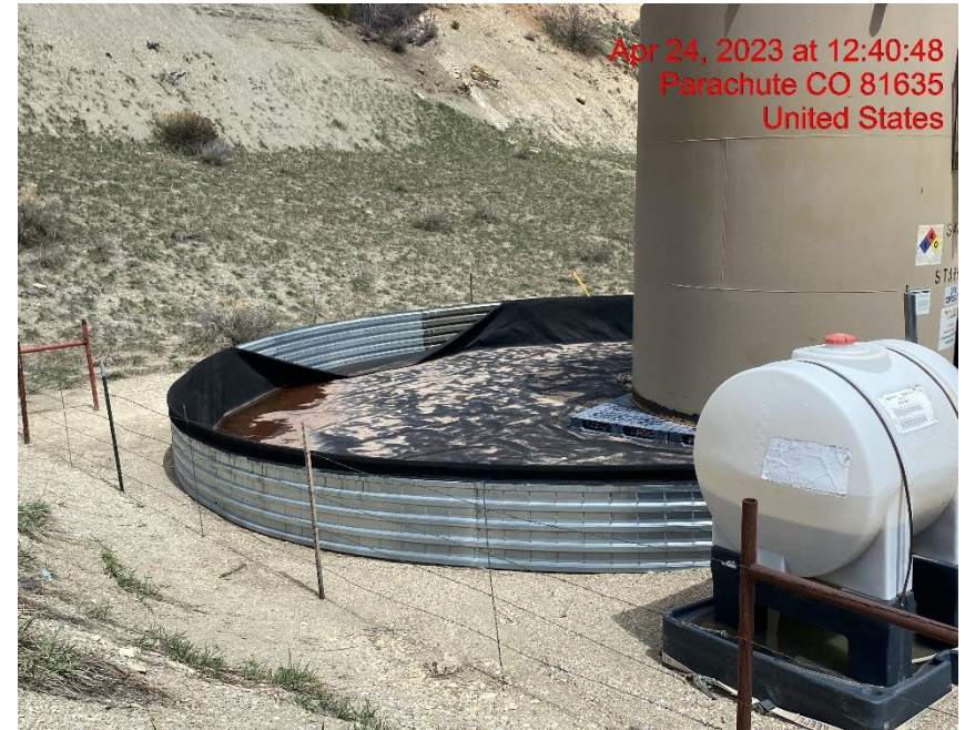
Berm Liner Damaged – Photo #02469
