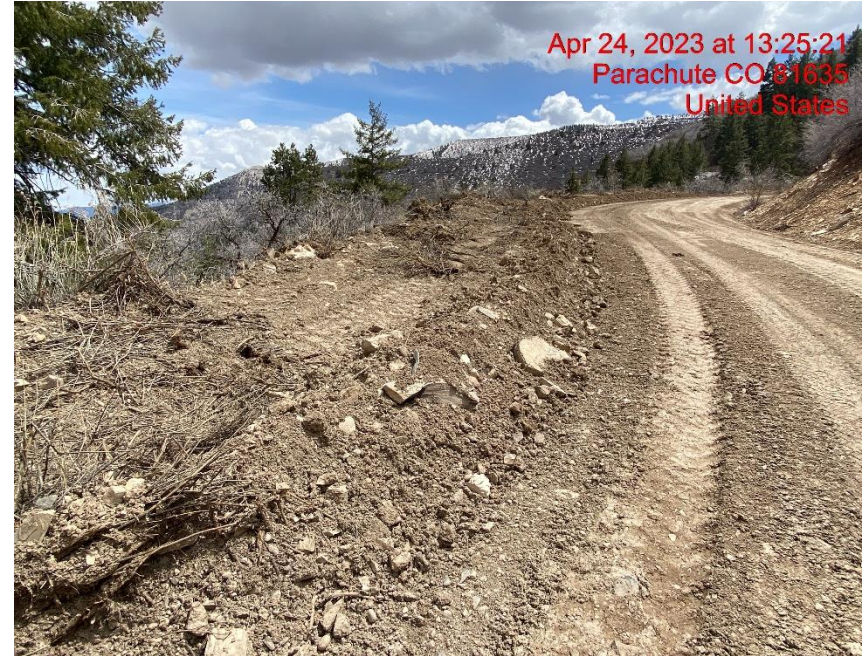
Access Road Degradation/Transportation of Sediment – Photo #02493
