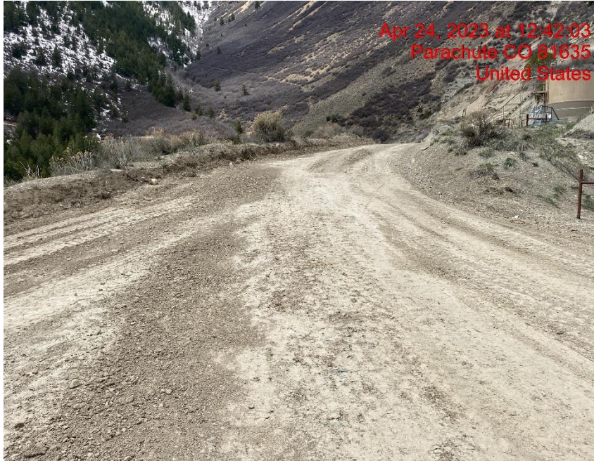
Inadequate Vehicle Tracking BMP at Location Entrance – Photo #02473
