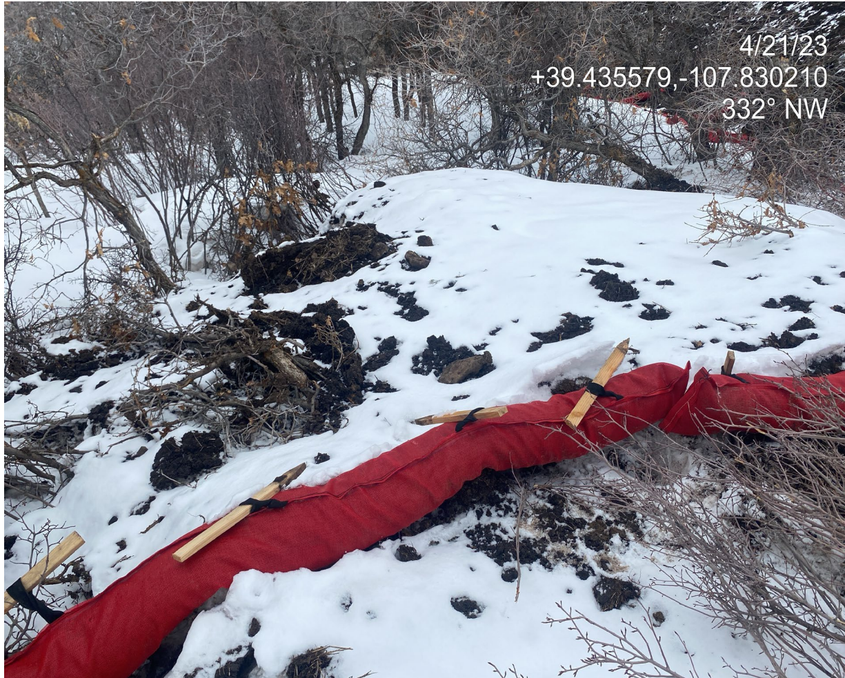
Photo 10. Photo shows perimeter stormwater BMPs at the west of the location are in disrepair.
