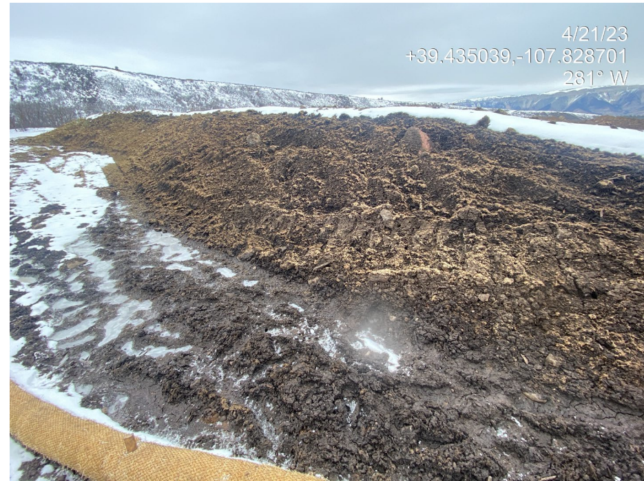
Photo 13. Photos show the topsoil stockpile at the south of the location. Hydromulch is not evenly distributed to cover the entire exposed soil surface. It appears mulch has not been applied from multiple angles to prevent shadow.
