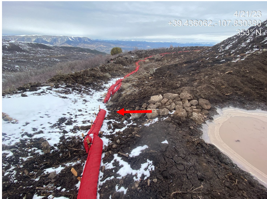
Photo 15. Photos show sediment traps at the northwest (left) and southwest (right). The outlets are designed to discharge stormwater directly into an unvegetated, unstabilized topsoil berm.
