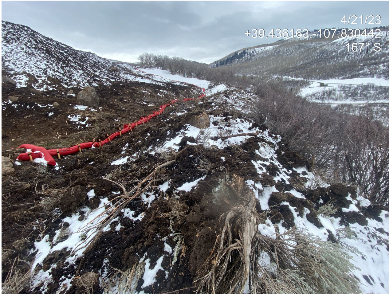
Photo 9. Photo taken from the west shows a lack of stormwater and topsoil protection BMPs. Topsoil is loose and unconsolidated and susceptible to erosion.
