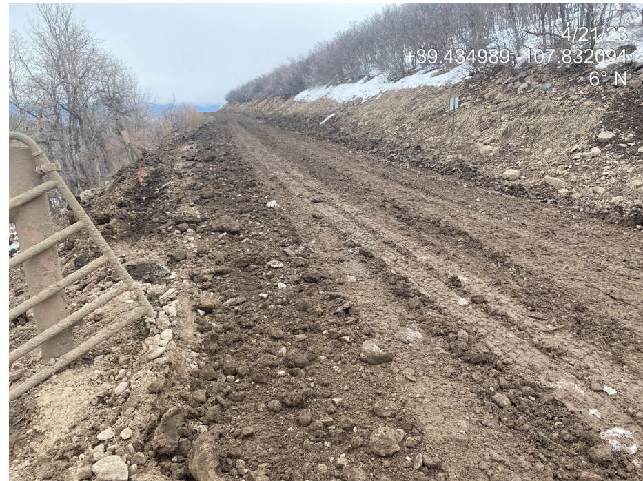
Photo 23. Photos show the location entrance (left) and the location access road (right) before it merges with county road 317. Tracking control BMPs are missing/insufficient.
