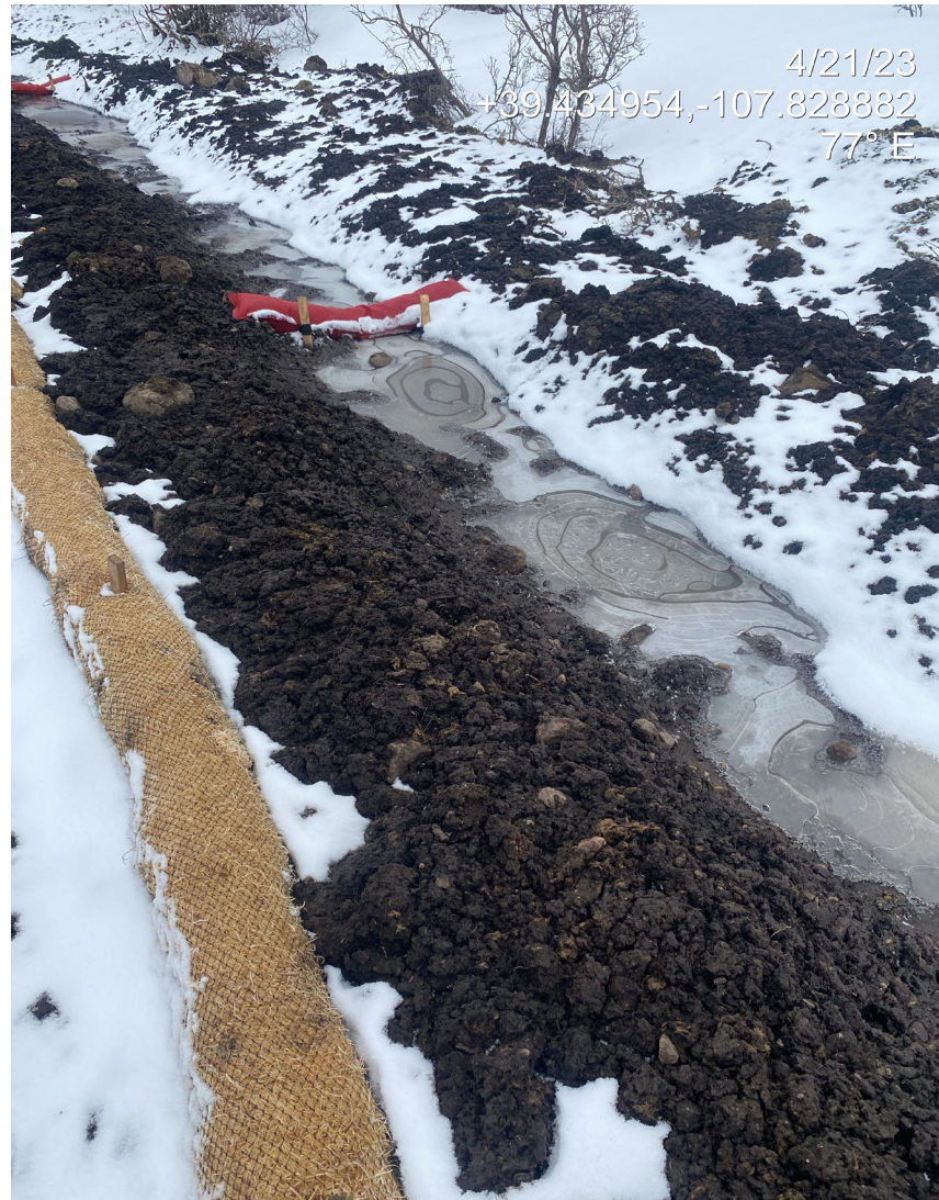
Photo 8. Photo taken from the south. Topsoil does not appear to have been salvaged. Stormwater BMPs appear to be constructed from topsoil.
