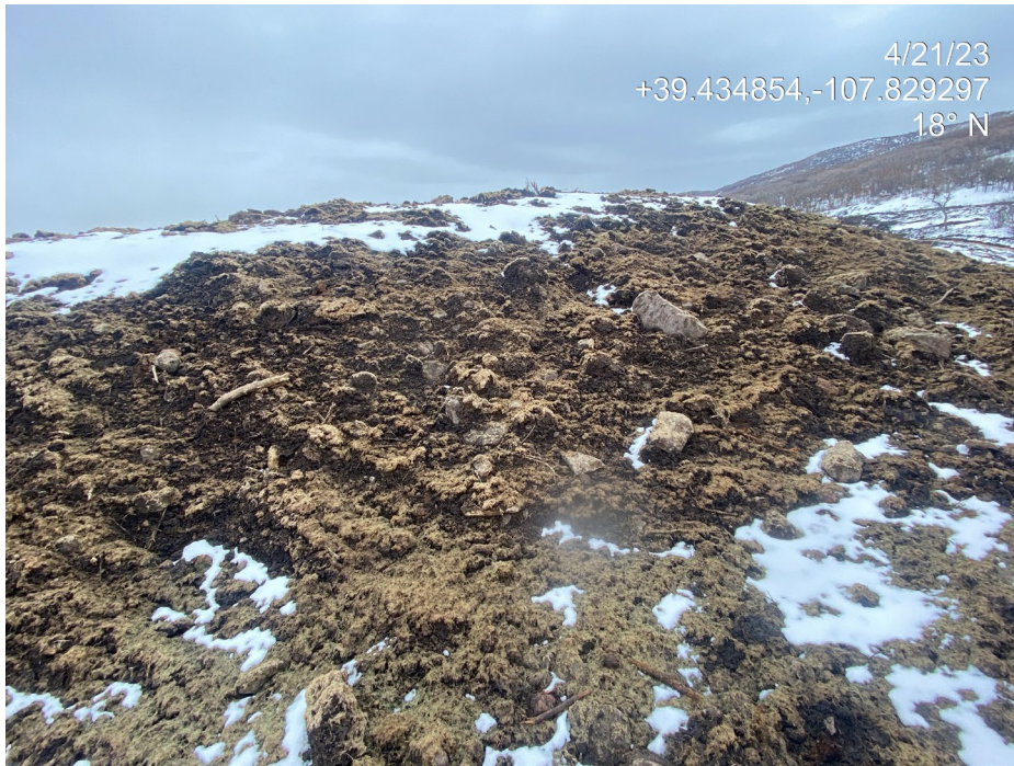
Photo 13. Photos show the topsoil stockpile at the south of the location. Hydromulch is not evenly distributed to cover the entire exposed soil surface. It appears mulch has not been applied from multiple angles to prevent shadow.
