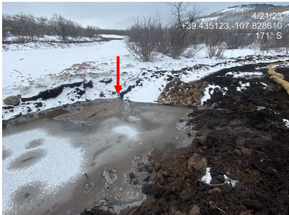
Photo 16. Photo taken from the southeast shows degradation where stormwater is bypassing an armored inlet to a sediment trap.
