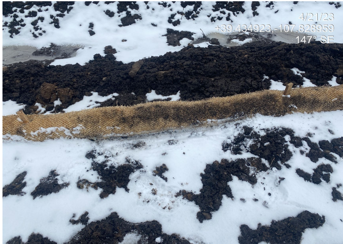
Photo 14. Photos show the topsoil stockpile at the south of the location. Some perimeter wattles are not installed in accordance with good engineering practices (trenched and backfilled).
