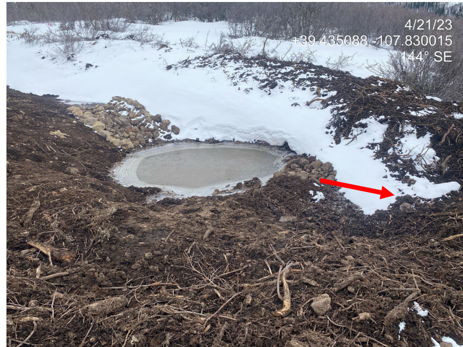
Photo 15. Photos show sediment traps at the northwest (left) and southwest (right). The outlets are designed to discharge stormwater directly into an unvegetated, unstabilized topsoil berm.
