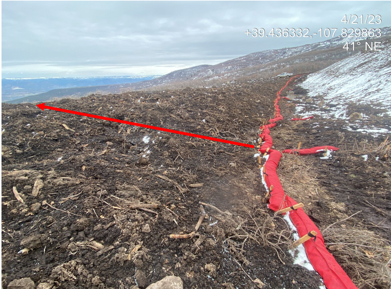
Photo 6. Photo taken from the north shows perimeter stormwater controls which are mapped at the northern edge of the location. The disturbance continues an additional ~70 feet to the north (red arrow).
