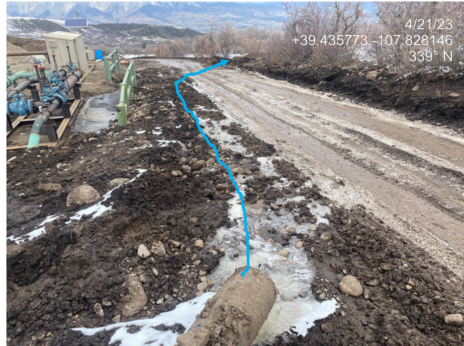
Photo 18. Photo taken from the east shows the stormwater pipe pictured in photo 17 is discharging concentrated stormwater flows without outlet protections. Stormwater is flowing down the access road where a water bar diverts it to the east of the access road without BMPs to manage flow or protect the discharge area.
