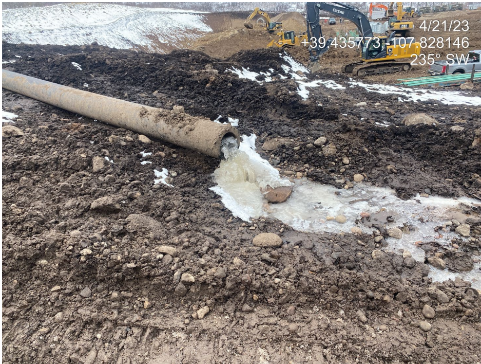
Photo 18. Photo taken from the east shows the stormwater pipe pictured in photo 17 is discharging concentrated stormwater flows without outlet protections. Stormwater is flowing down the access road where a water bar diverts it to the east of the access road without BMPs to manage flow or protect the discharge area.
