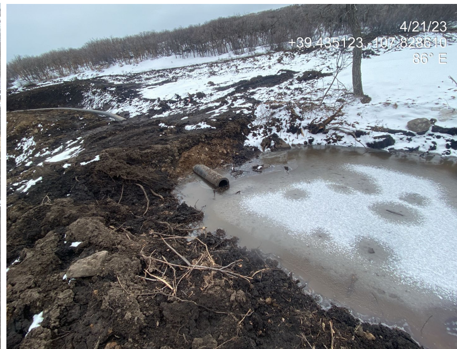
Photo 17. Photo shows the outlet pipe for the sediment trap pictured in Photo 16.
