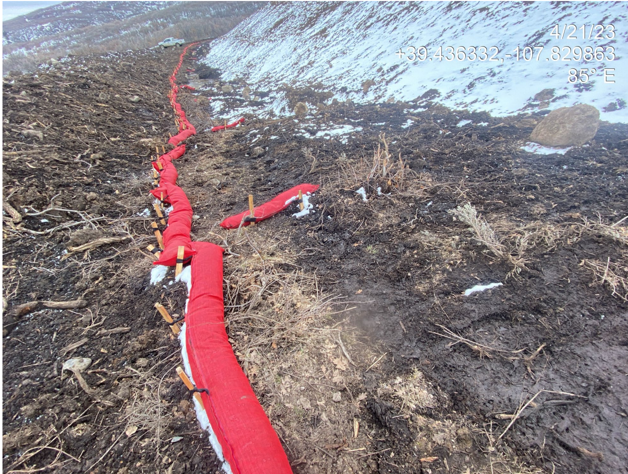
Photo 7. Photo taken from the north. Topsoil does not appear to have been salvaged at stormwater BMPs (note dark soil color and presence of vegetation). Photo also shows the diversion ditch has not been properly constructed per good engineering practices.
