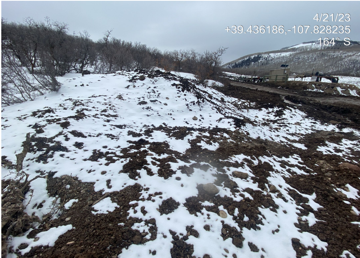
Photo 20. Refer to Photo 18 comment. Concentrated stormwater flows are being discharged into a loose, unconsolidated pile of soil to the east of the access road.
