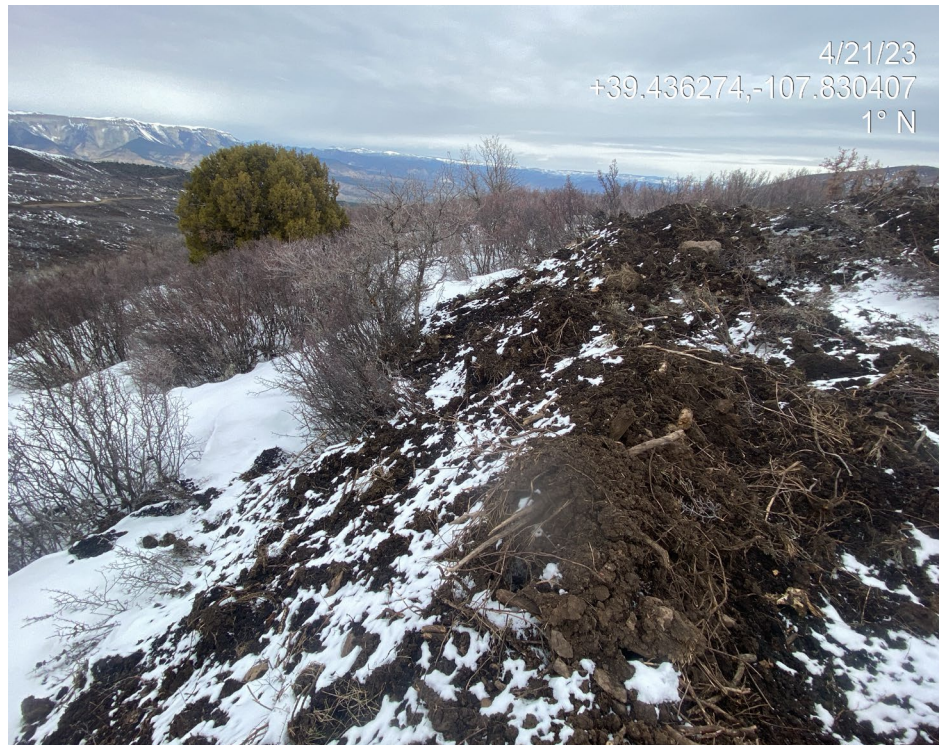
Photo 4. Photo taken from the northwestern edge of the location shows “LOD 1” from Photo 3. Note also lack of protections for unconsolidated topsoil subject to erosion.
