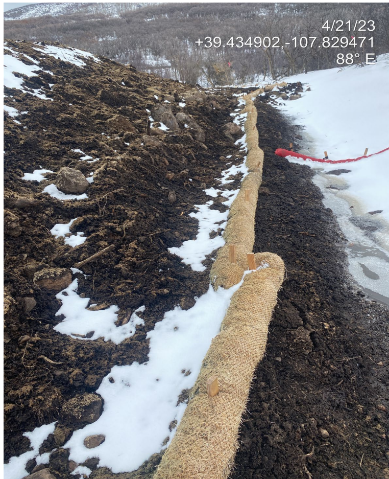
Photo 14. Photos show the topsoil stockpile at the south of the location. Some perimeter wattles are not installed in accordance with good engineering practices (trenched and backfilled).
