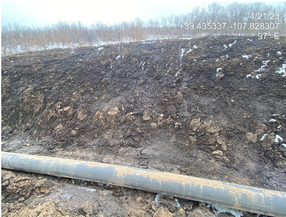
Photo 21. Photo taken from the south shows rill erosion occurring on bare, unprotected, unstabilized slopes.
