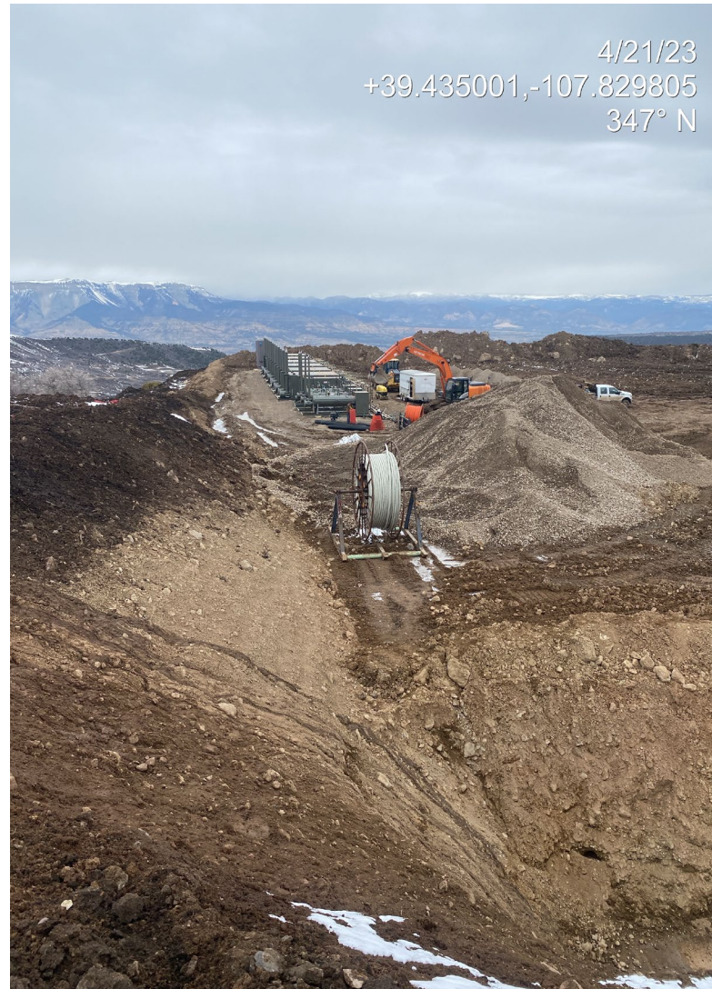
Photo 12. Photo taken from the southwest shows topsoil (darker colored) is unstabilized and eroding. BMPs to stabilize and protect topsoil are missing/insufficient.
