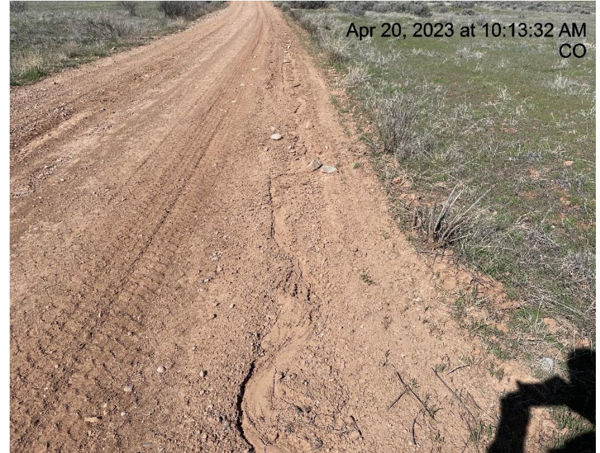
Photo # 5876 Erosion & transport of sediment down spur road
