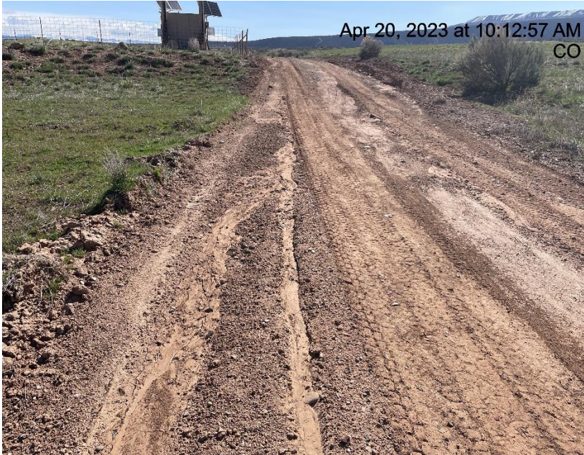
Photo # 5875 Erosion & transport of sediment down spur road
