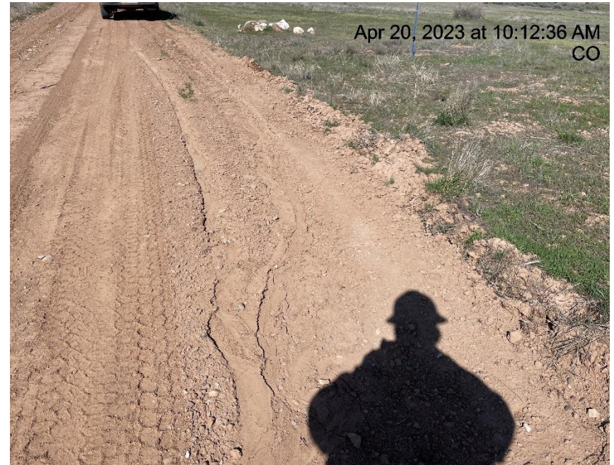
Photo # 5874 Erosion & transport of sediment down spur road
