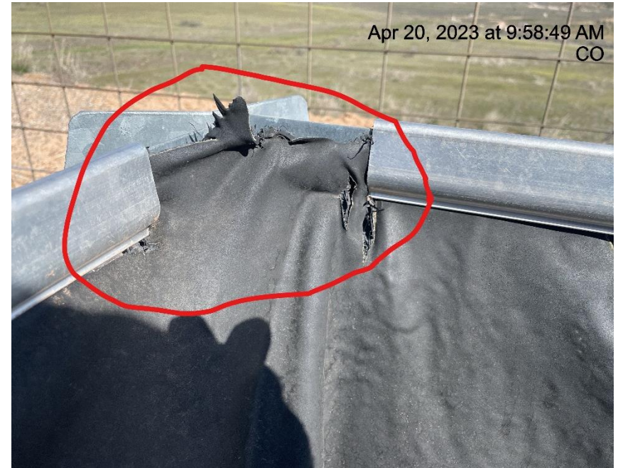
Photo # 5846 Containment liner needs maintenance
