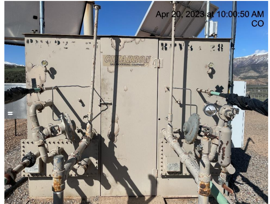
Photo # 5852 Meter calibration info not conspicuously posted
