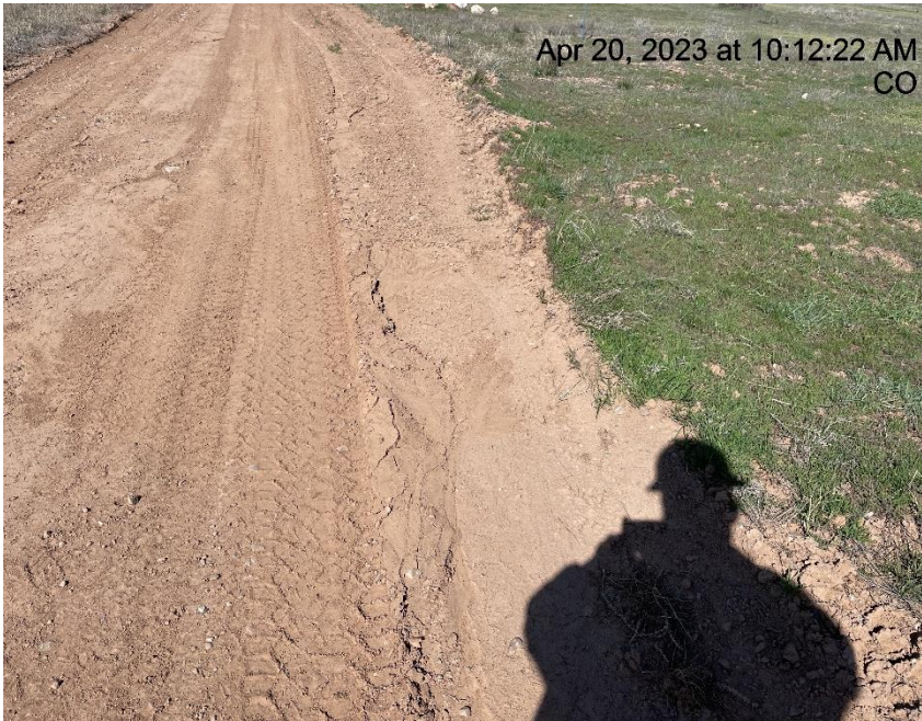
Photo # 5873 Erosion & transport of sediment down spur road
