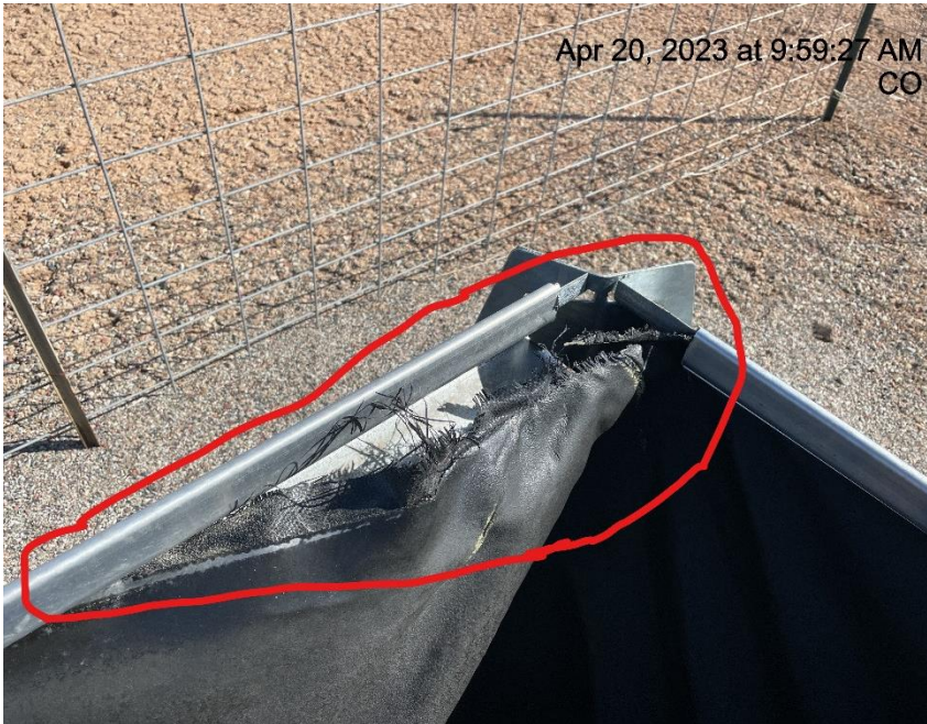
Photo # 5849 Containment liner needs maintenance
