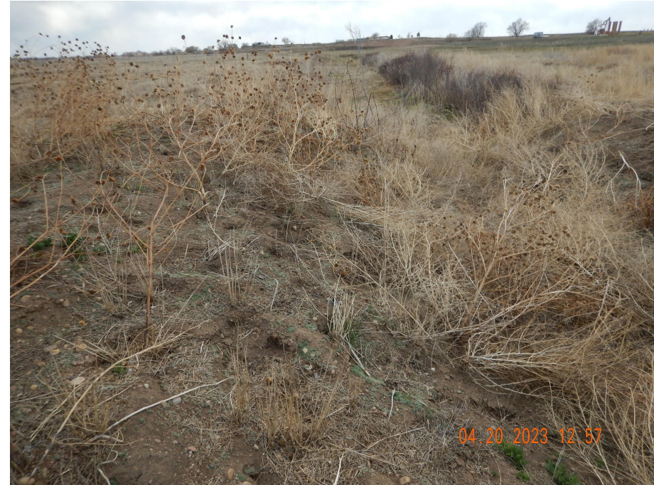
Photo 7. Photo taken from the southern drainage crossing, facing South. This area needs to be recontoured as the bottom is higher than the drainage which could impede flow.
