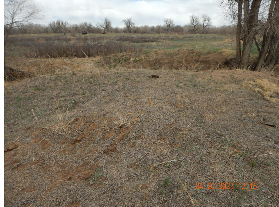
Photo 5. Photo taken from the northern drainage crossing, facing North. This area needs to be recontoured as the bottom is higher than the drainage which could impede flow.
