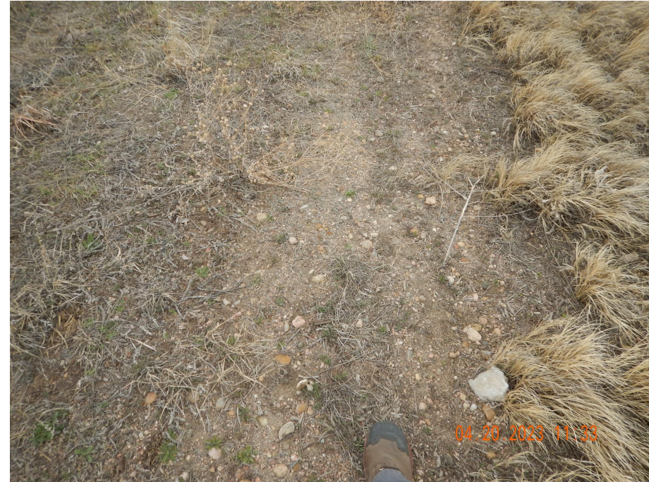
Photo 3. Close up photo taken from a portion of the access road. It does not appear all the gravel has been removed.
