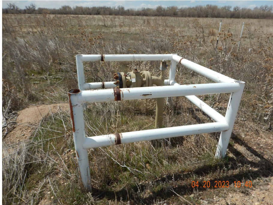
Photo 9. Photo taken from the offsite tank battery location, facing South. Photo illustrates what appears to be unused midstream equipment. Operator shall coordinate with the midstream Operator to get this removed.
