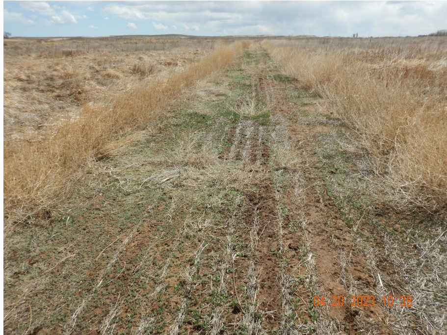
Photo 5. Photo taken along a section of the access road, facing East. Photo illustrates weedy establishment and weed debris growing along the access road.
