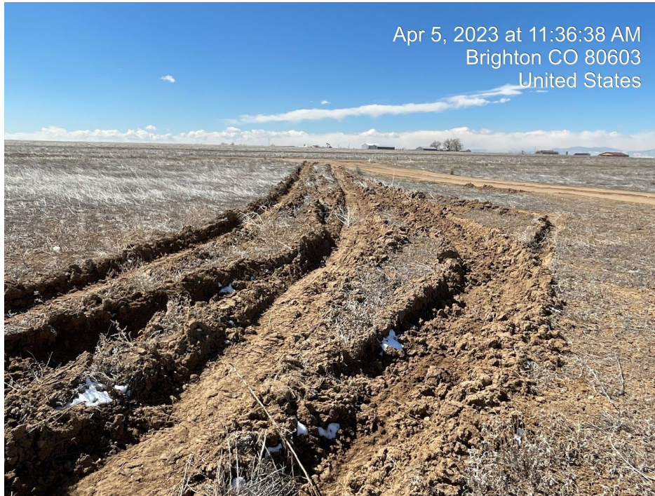
Photo 4. Photo taken of disturbance out of designated area, deep ruts caused by equipment.
