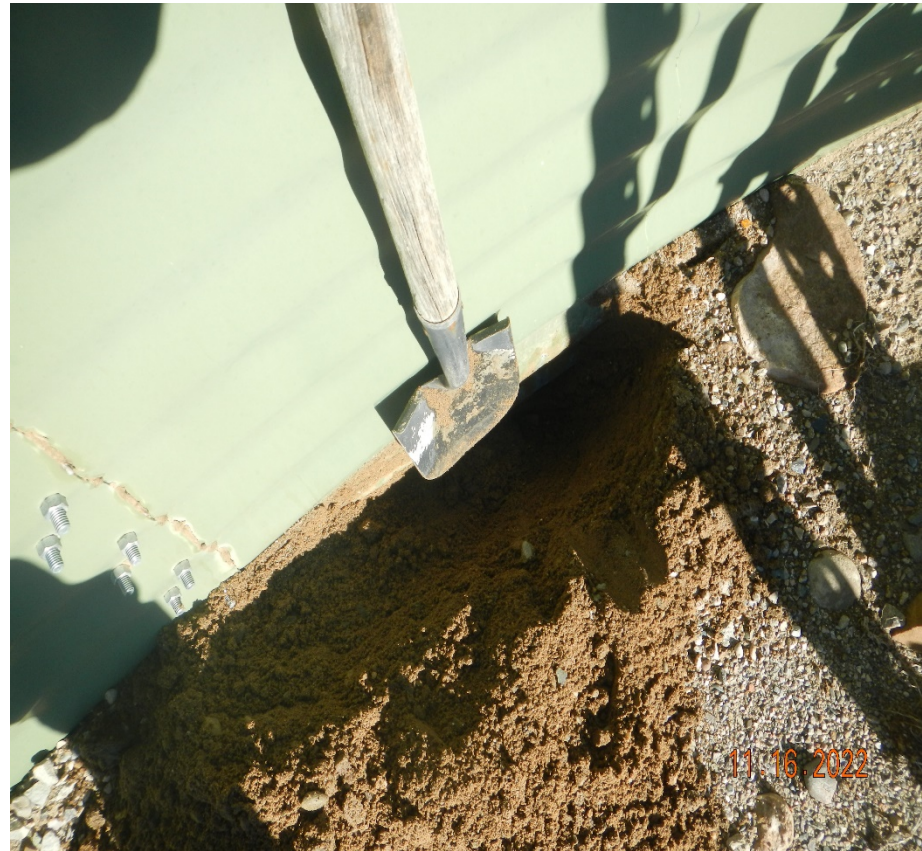
Photo 5. The steel containment is only about 4 inches below grade. The steel containment is not constructed per the Operator's SWMP.
