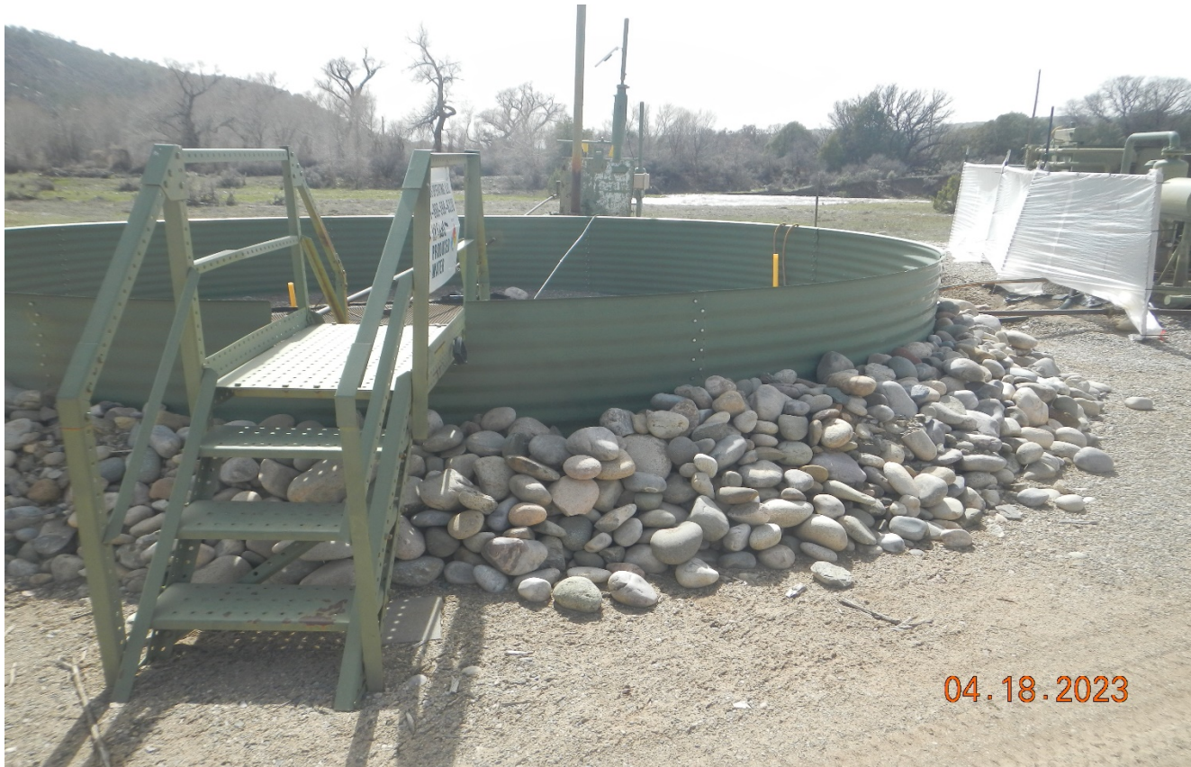
Photo 3. Facing toward the open top tank. There is round rock placed around the containment which will not prevent flood water from entering underneath the steel containment. The steel containment is not constructed per the Operator's SWMP. Previous corrective action has not been completed.
