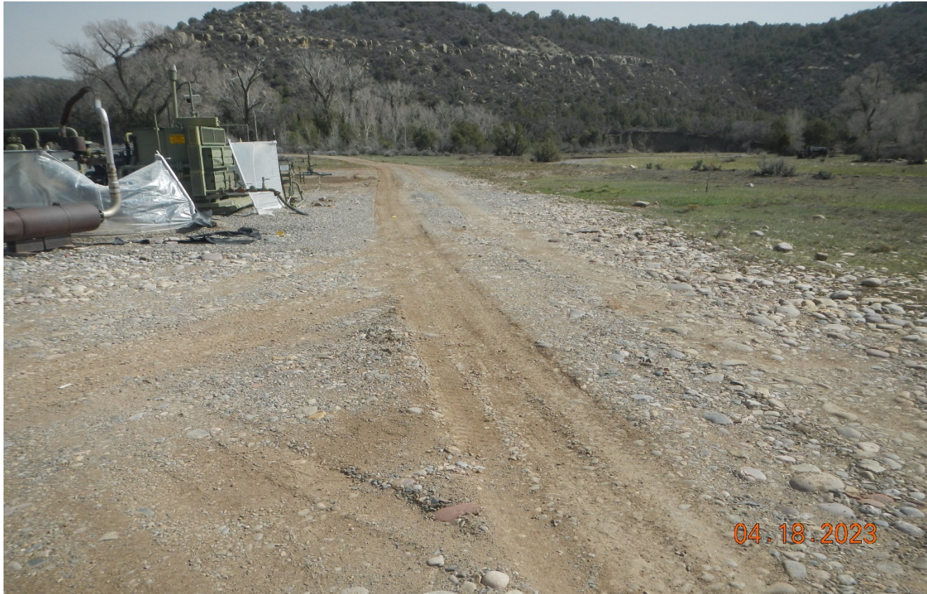
Photo 8. Facing southeast toward the location. The area of the road shows signs of scouring where flood flows across the road from left to right towards the Florida River.
