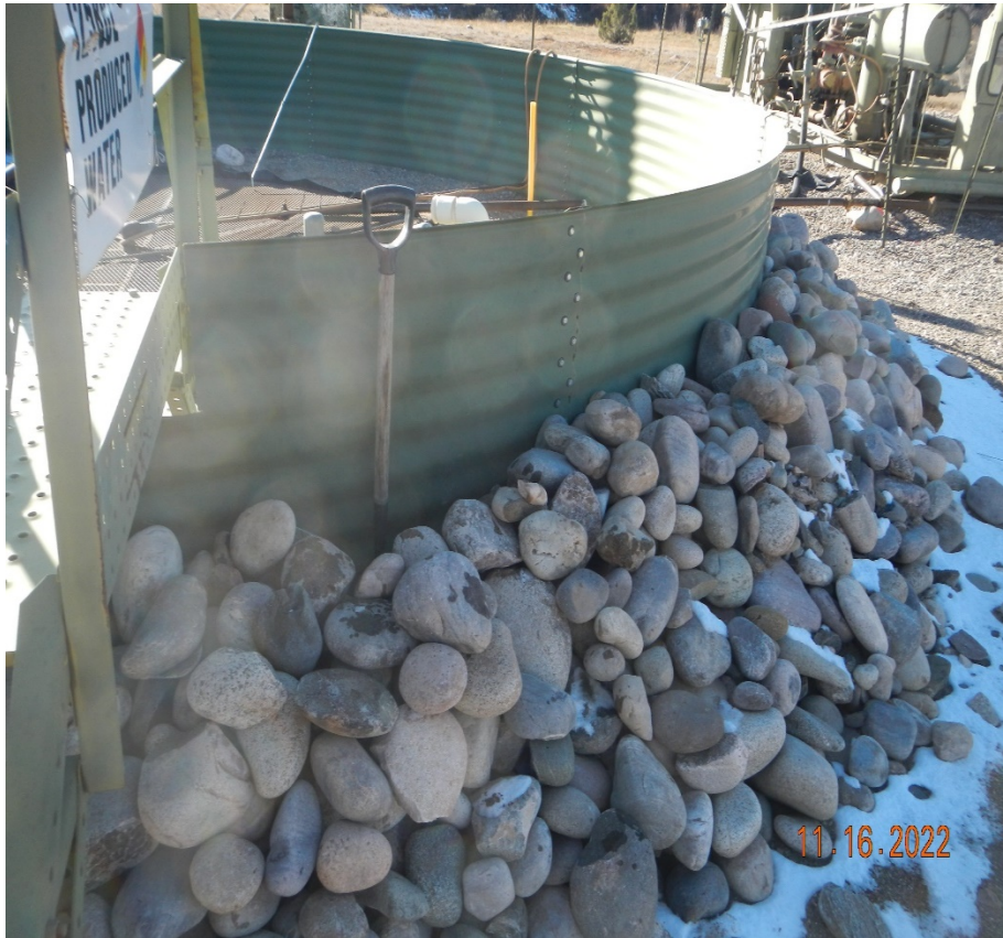
Photo 4. The steel containment is no constructed per the Operator's SWMP. A 3.5 ft. shovel was placed at the containment for scale.
