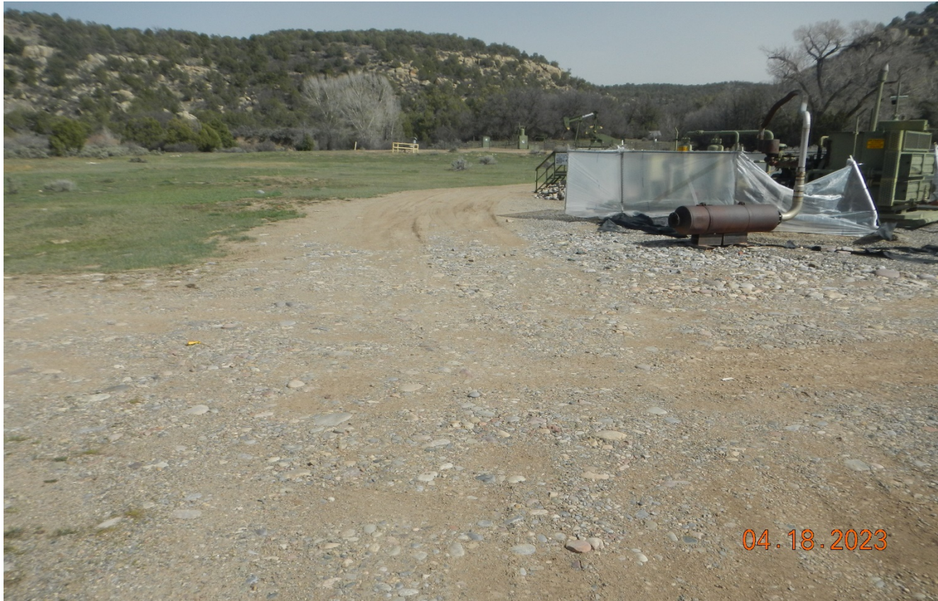
Photo 9. Facing southeast toward the location. The area of the road shows signs of scouring where flood flows across the road from left to right towards the Florida River.
