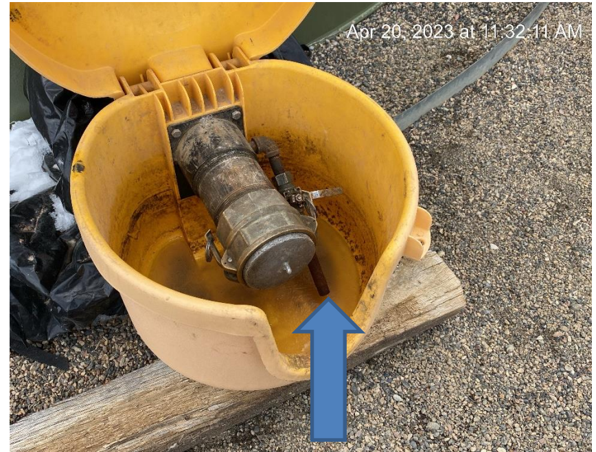
Open end valve on loadline
