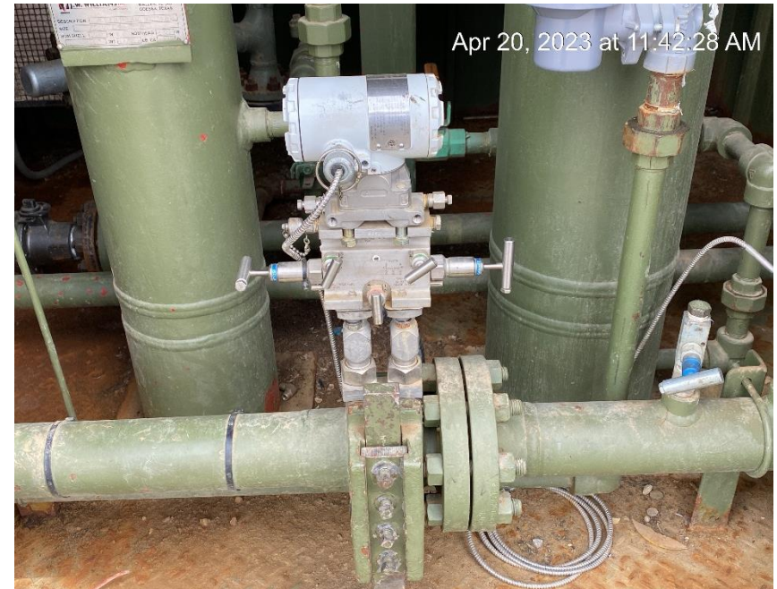
Last gas meter calibration date not posted
