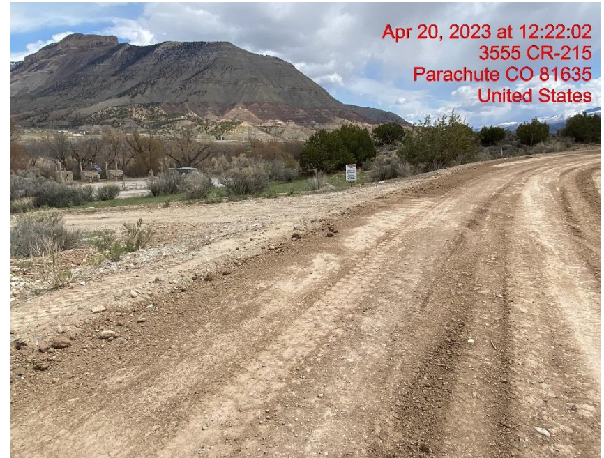
Inadequate Vehicle Tracking BMP at Location Entrance/Exit – Photo #02418
