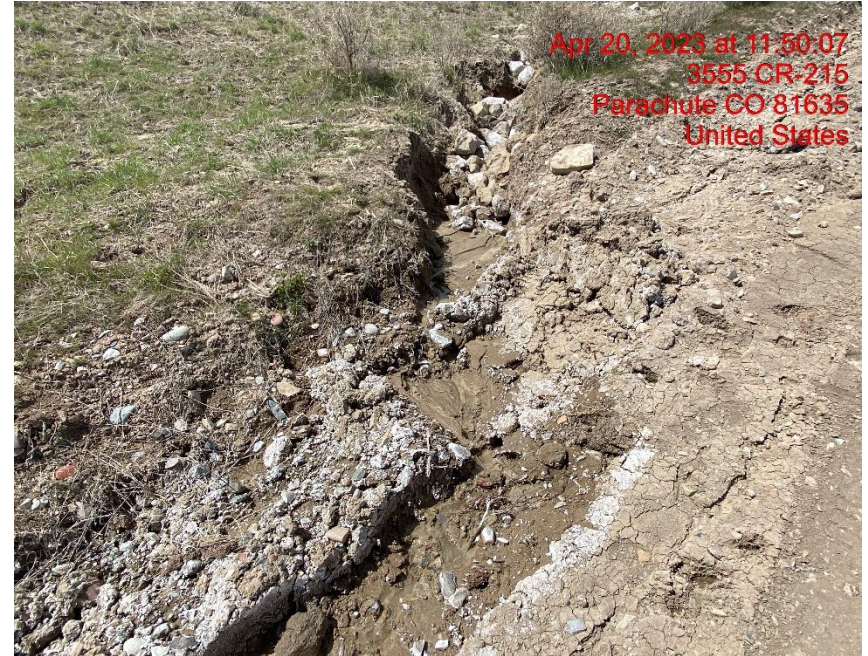
Access Road Ditch Erosion– Photo #02395
