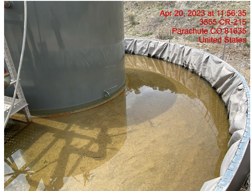
Inadequate Berm Capacity - Photo #02406
