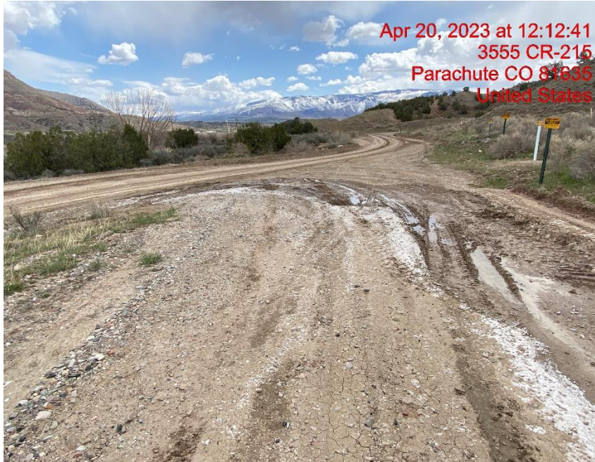
Inadequate Vehicle Tracking BMPs at Location Entrance/Exit – Photo #02409
