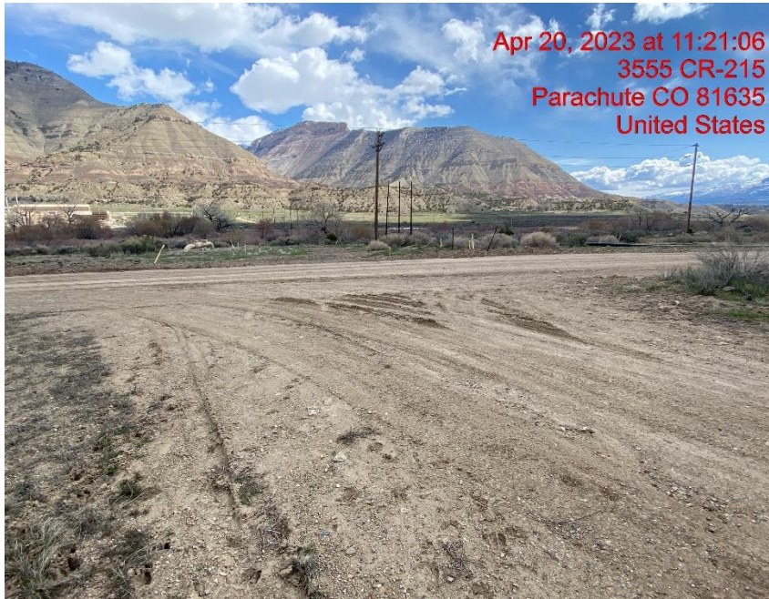
Inadequate Vehicle Tracking BMP at Location Entrance/Exit – Photo #02383
