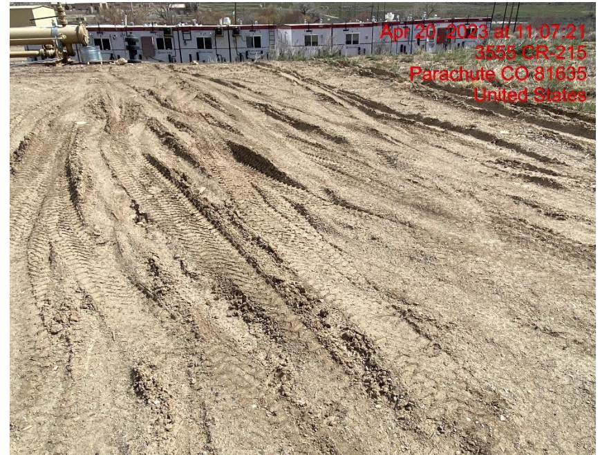
Lack of Stabilization – Photo #02381
