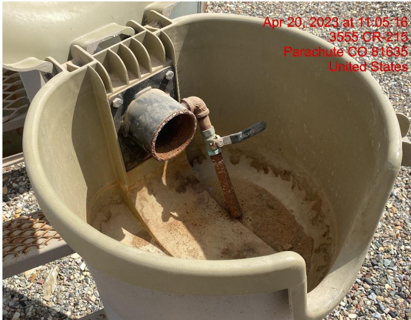
Open-Ended Load Line – Photo #02378
