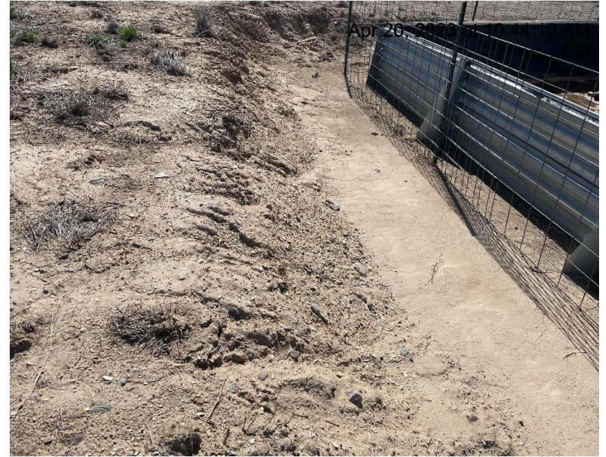
Photo # 5915 Erosion & Transport of sediment/Sediment encroaching on equipment
