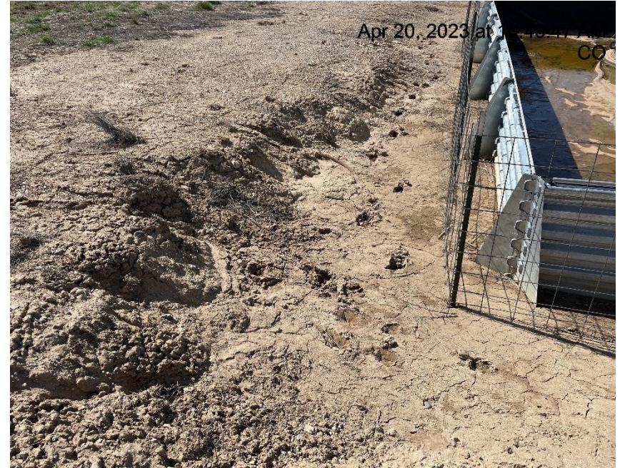
Photo # 5913 Erosion & Transport of sediment/Sediment encroaching on equipment
