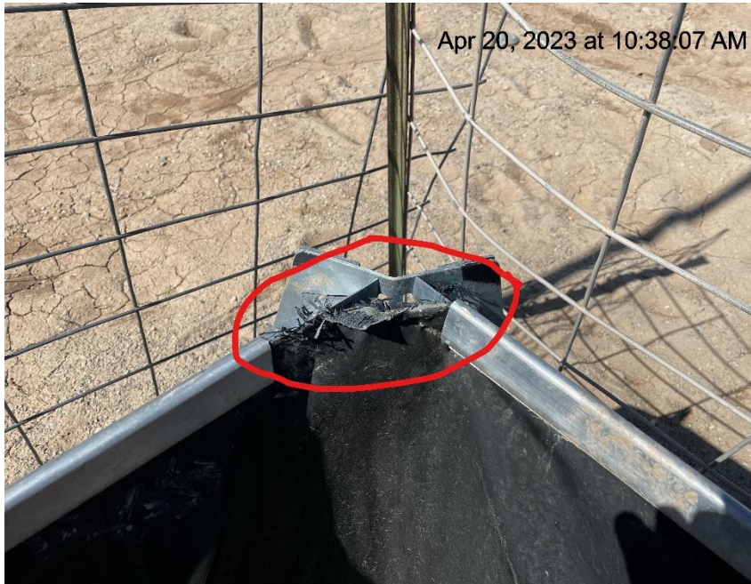
Photo # 5901 Containment liner needs maintenance
