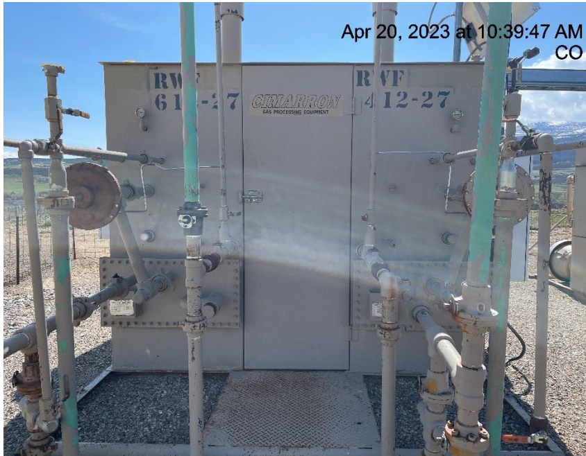
Photo # 5904 Meter calibration info not conspicuously posted
