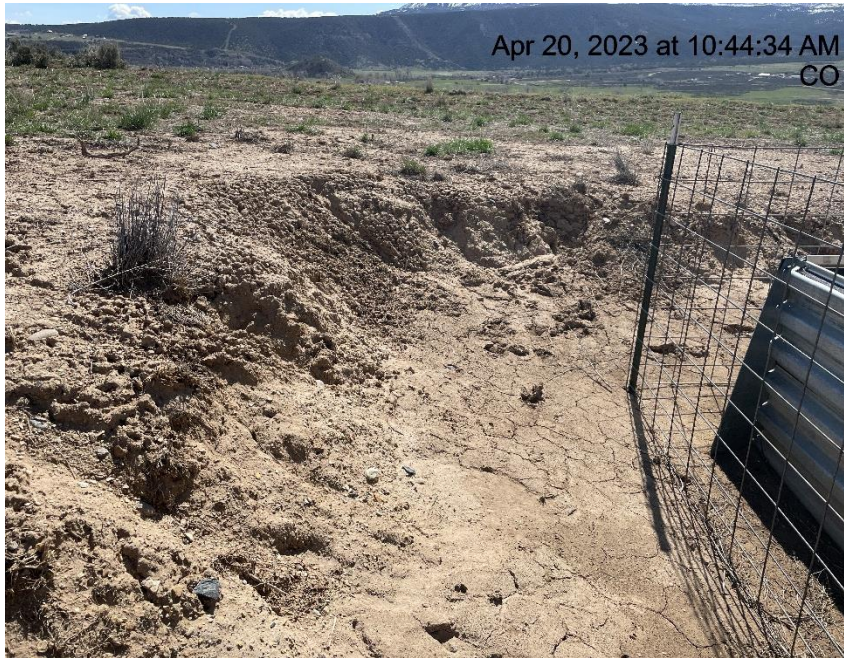
Photo # 5919 Erosion & Transport of sediment/Sediment encroaching on equipment
