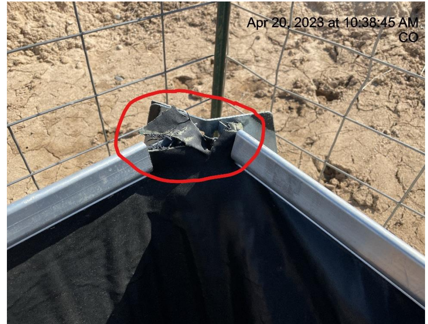
Photo # 5902 Containment liner needs maintenance
