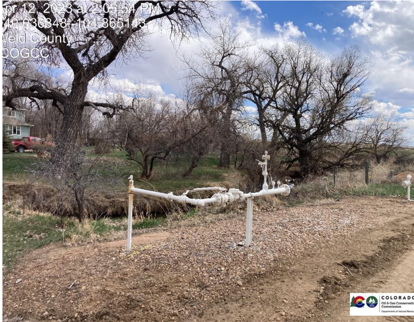
Pic 3 Gas meter run has been removed
