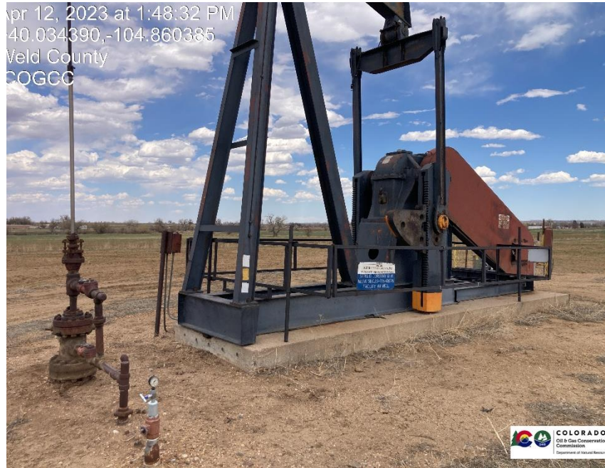
Pic 1 wellhead / pump jack
