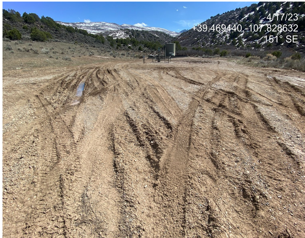
Photo 3. Photos show lack of stabilization of the working pad.
