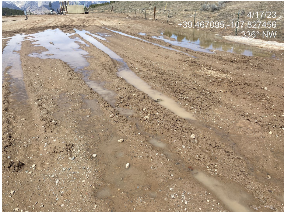
Photo 5. Photos show lack of stabilization of the working pad.
