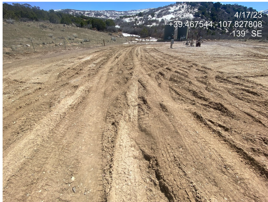
Photo 4. Photo shows lack of stabilization of the working pad.
