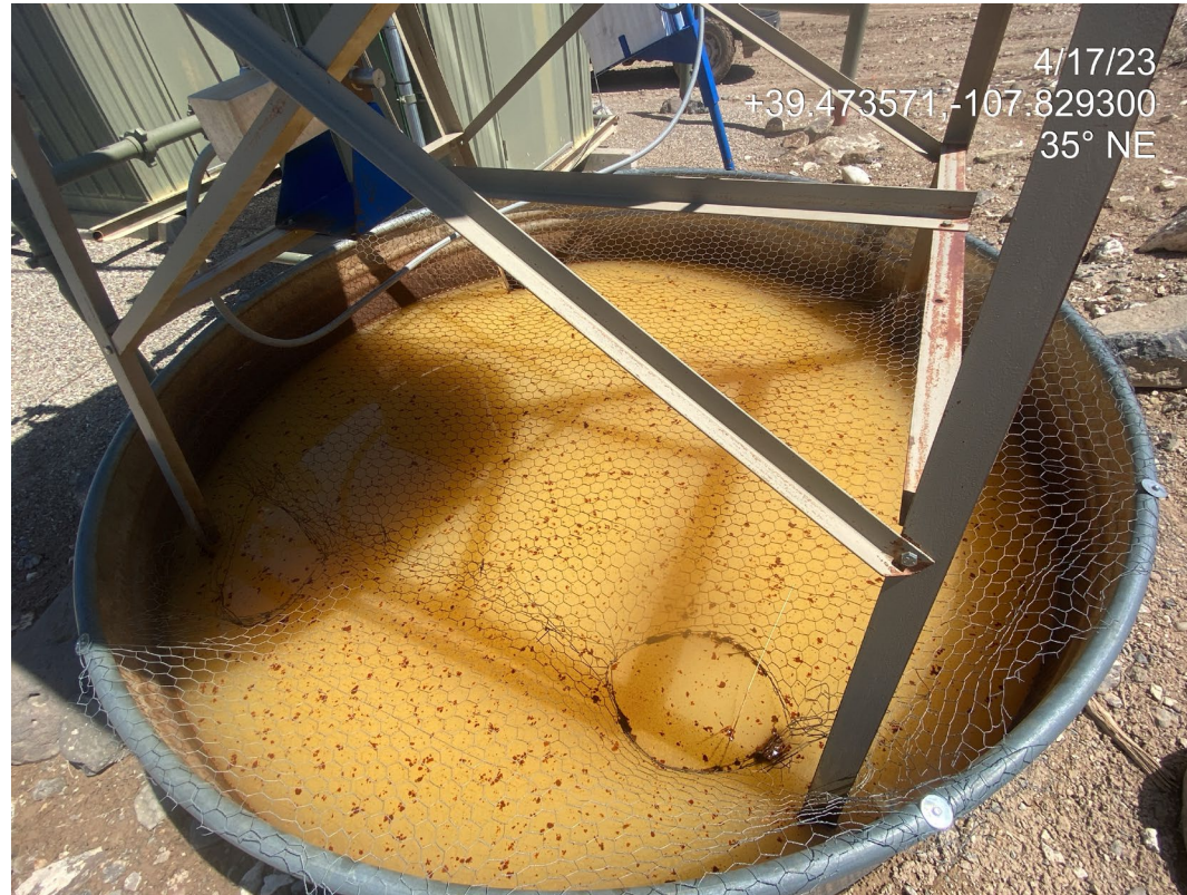
Photo 2. Photos show impacted fluid within the methanol tank secondary containment. Photos also show the wire mesh wildlife protection BMP has holes in it.
