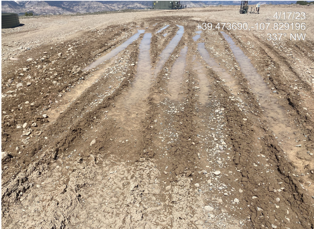
Photo 5. Photo shows lack of stabilization of a portion of the working pad area.
