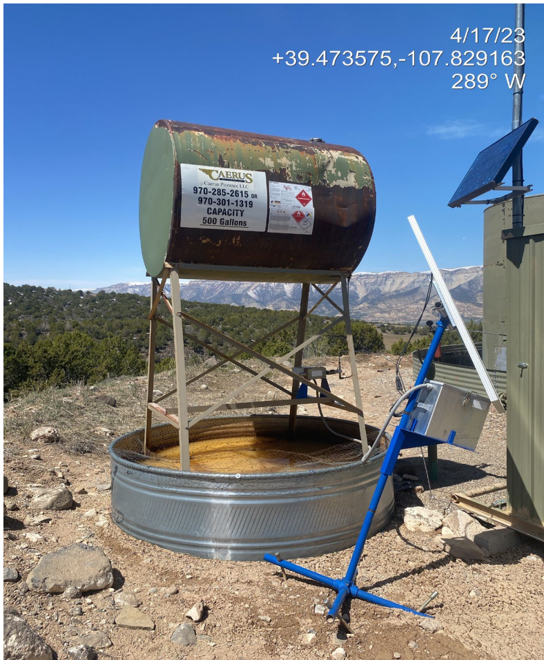
Photo 2. Photos show impacted fluid within the methanol tank secondary containment. Photos also show the wire mesh wildlife protection BMP has holes in it.
