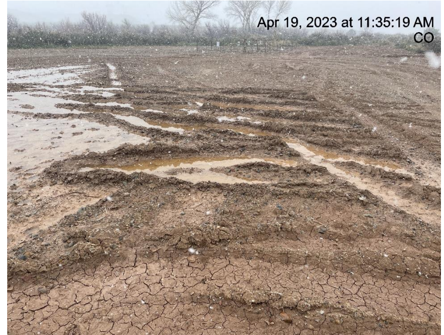
Photo # 5771 Lack of stabilization/compaction
