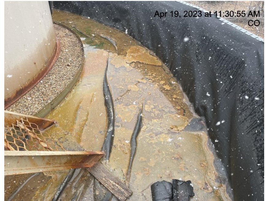
Photo # 5758 E & P waste is secondary containment
