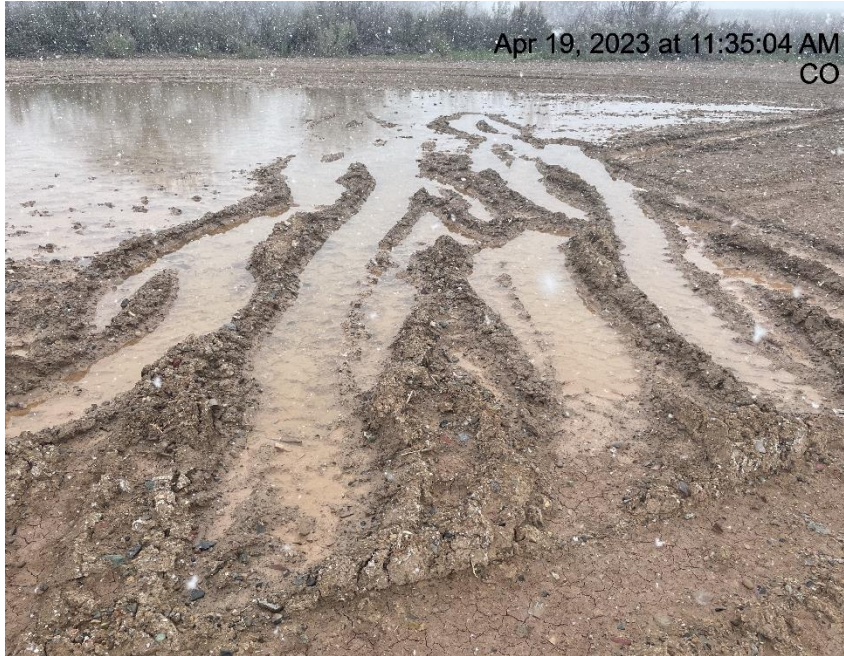
Photo # 5770 Lack of stabilization/compaction
