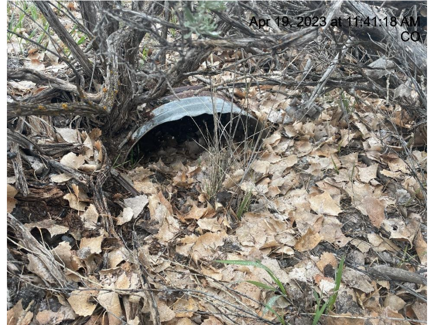
Photo # 5784 Culvert needs maintenance (on lease road near entrance to location)
