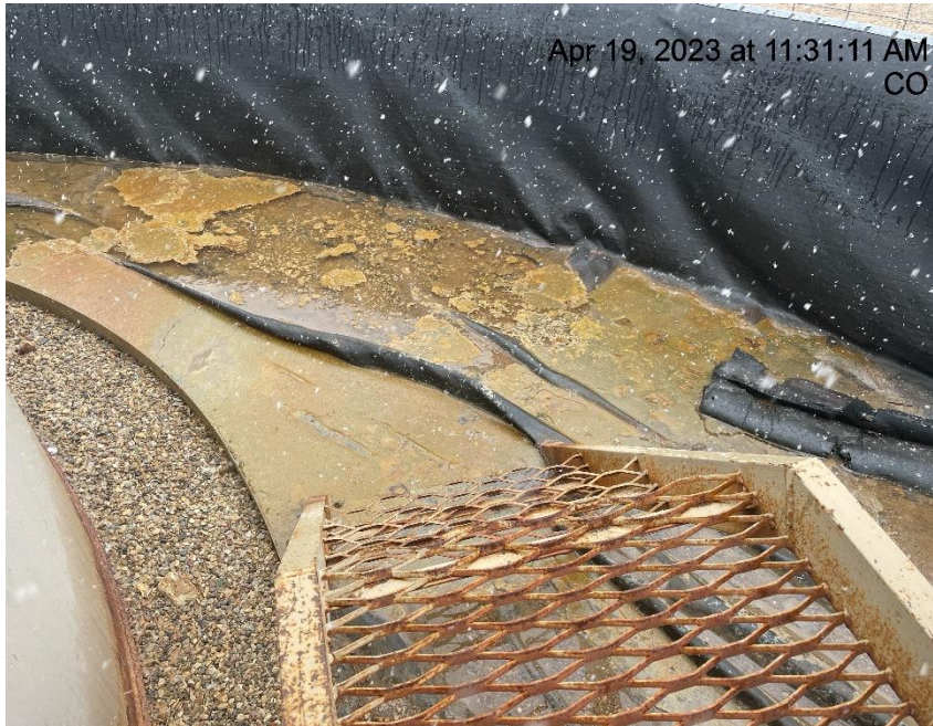
Photo # 5760 E & P waste is secondary containment
