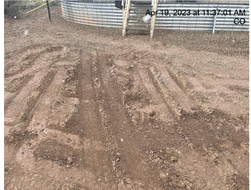
Photo # 5776 Lack of stabilization/compaction
