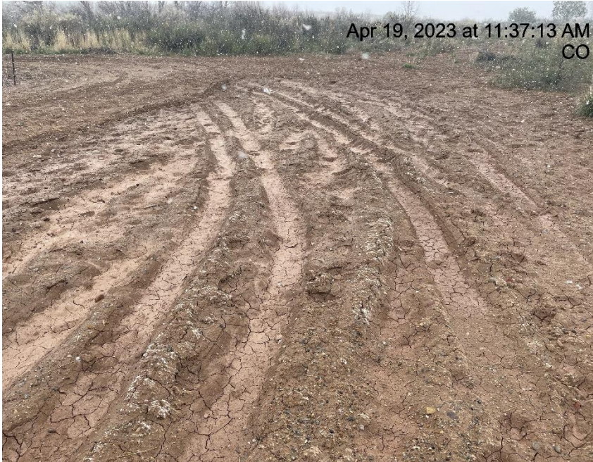
Photo # 5777 Lack of stabilization/compaction
