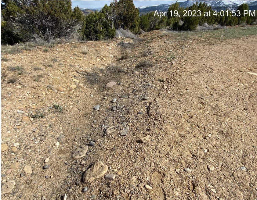
Direct drainage off location. No check dams or sediment trap.
