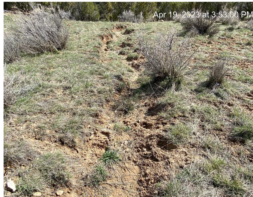
Direct drainage off location. No check dam or sediment trap.
