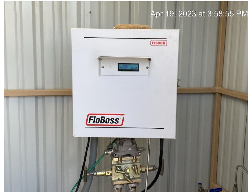
Gas meter calibration not visibly displayed
