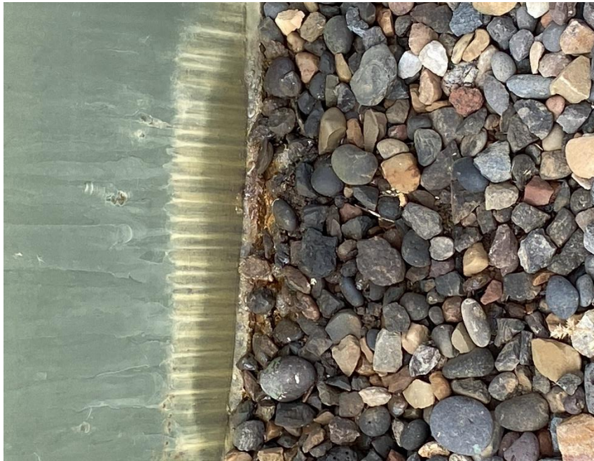
Soil staining inside tank battery
