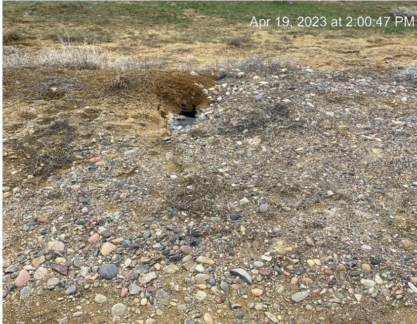
Erosion and sediment migration leaving location
