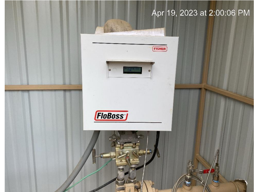
Gas meter calibration card not visibly displayed
