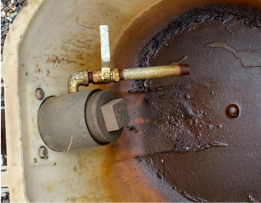
Drain valve on loadline lacks cap or plug
