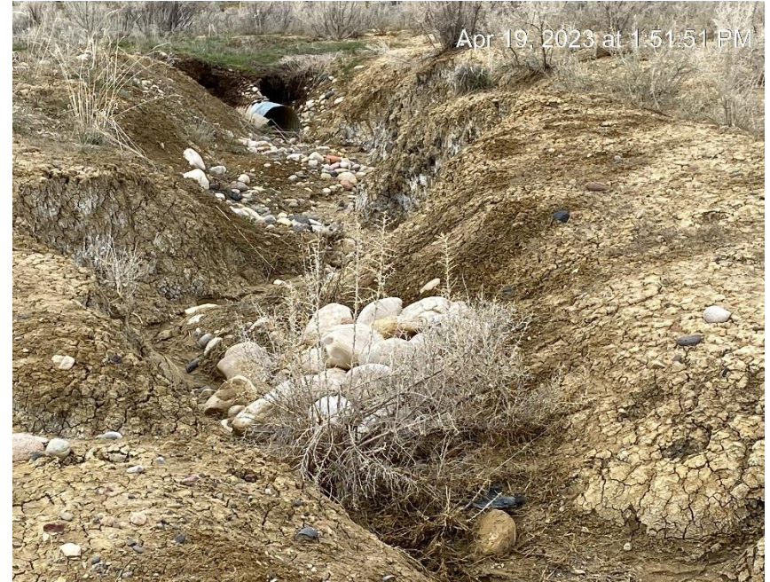
Check dams and culvert erosion
