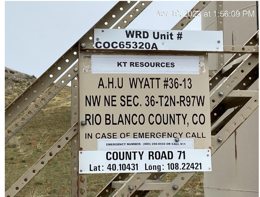
API Number missing from tank battery sign
