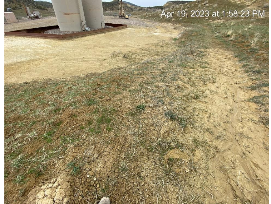
Bypass ditch full of sediment, erosion and sediment migration entering location
