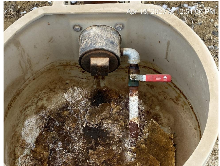
Drain valve has no cap or plug
