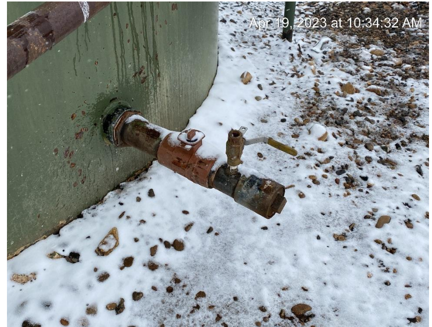
Valve lacking plug
