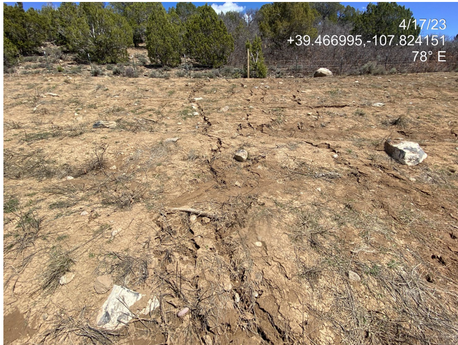
Photo 7. Photos show interim area slopes at the east are unstabilized.
