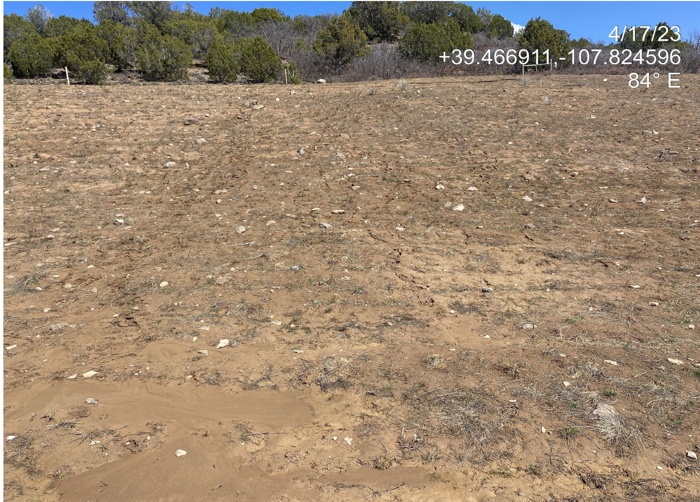
Photo 6. Photos show interim area slopes at the east are unstabilized.
