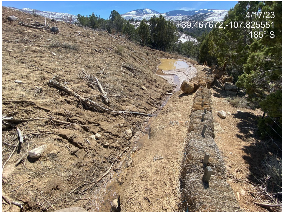
Photo 13. Photos show BMPs at the west of the location including erosion of the sediment trap walls.
