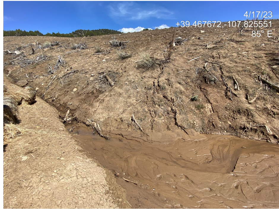
Photo 13. Photos show BMPs at the west of the location including erosion of the sediment trap walls.
