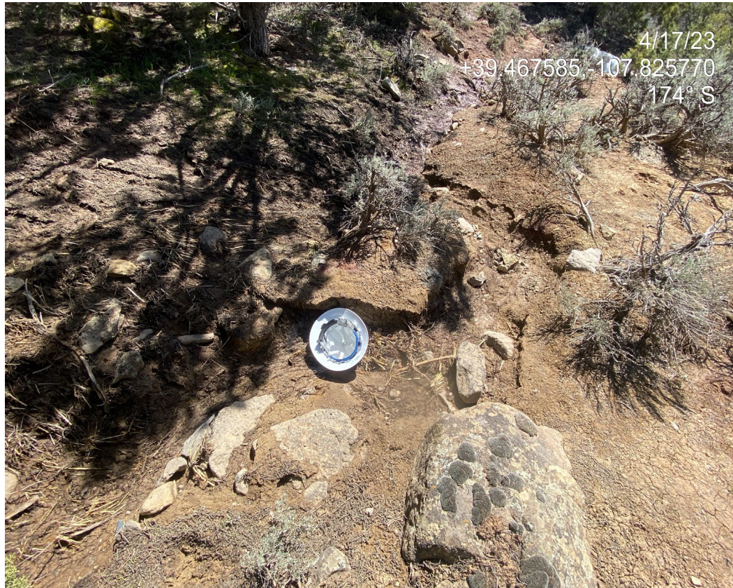
Photo 15. Photos show offsite degradation downslope of the sediment trap outlet pictured in Photo 13.
