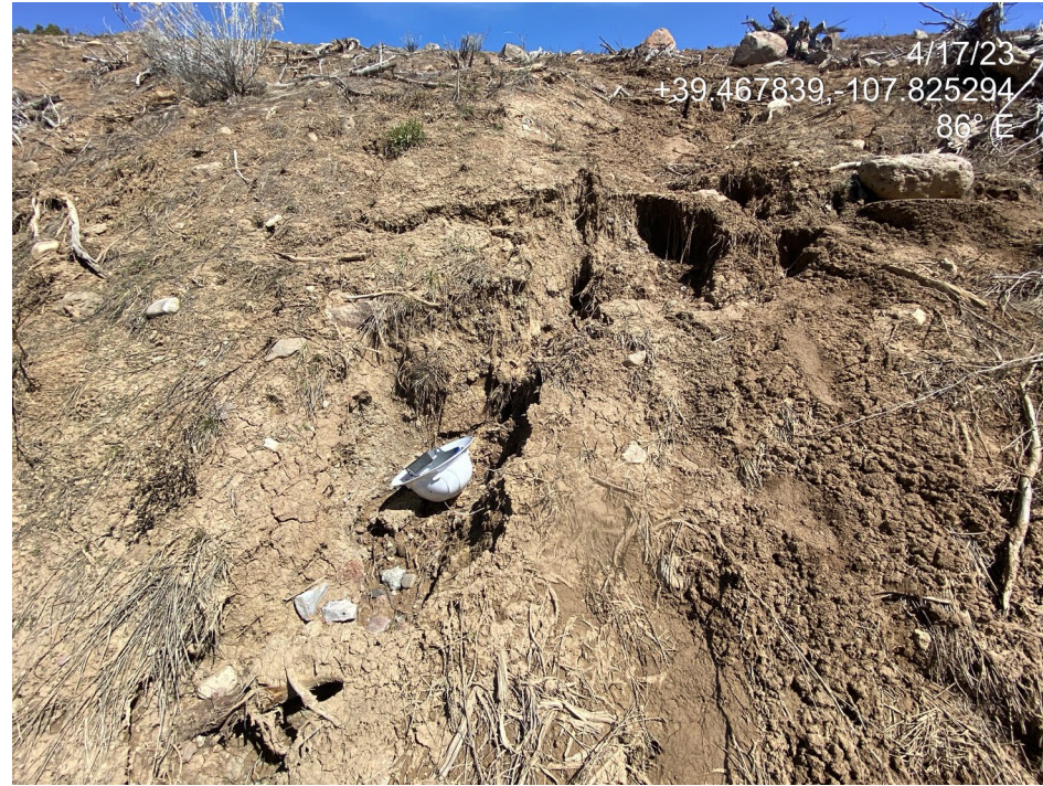
Photo 12. Photos show a sediment trap at the northwest of the location. The interim area above and side of the trap is not stabilized.
