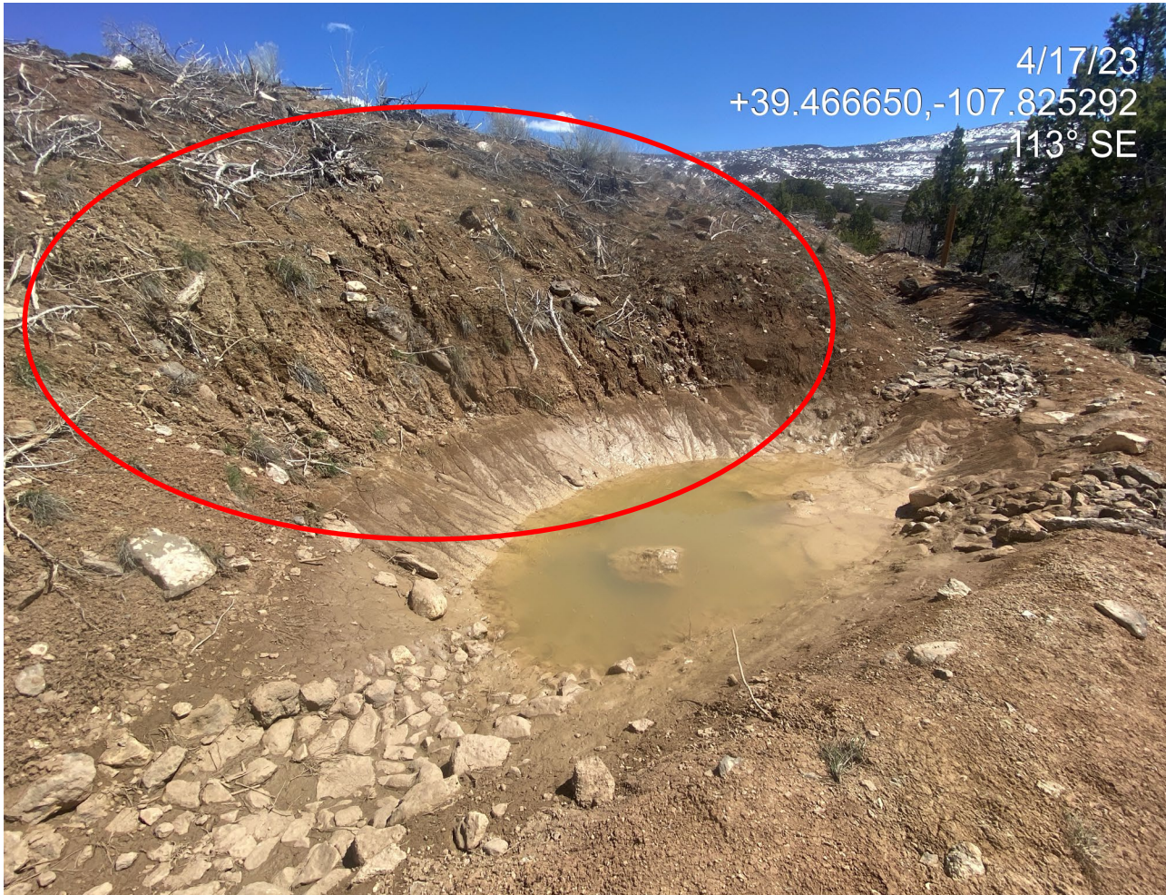
Photo 11. Photo shows a sediment trap at the southwest of the location. The interim area above and the side of the trap are not stabilized.
