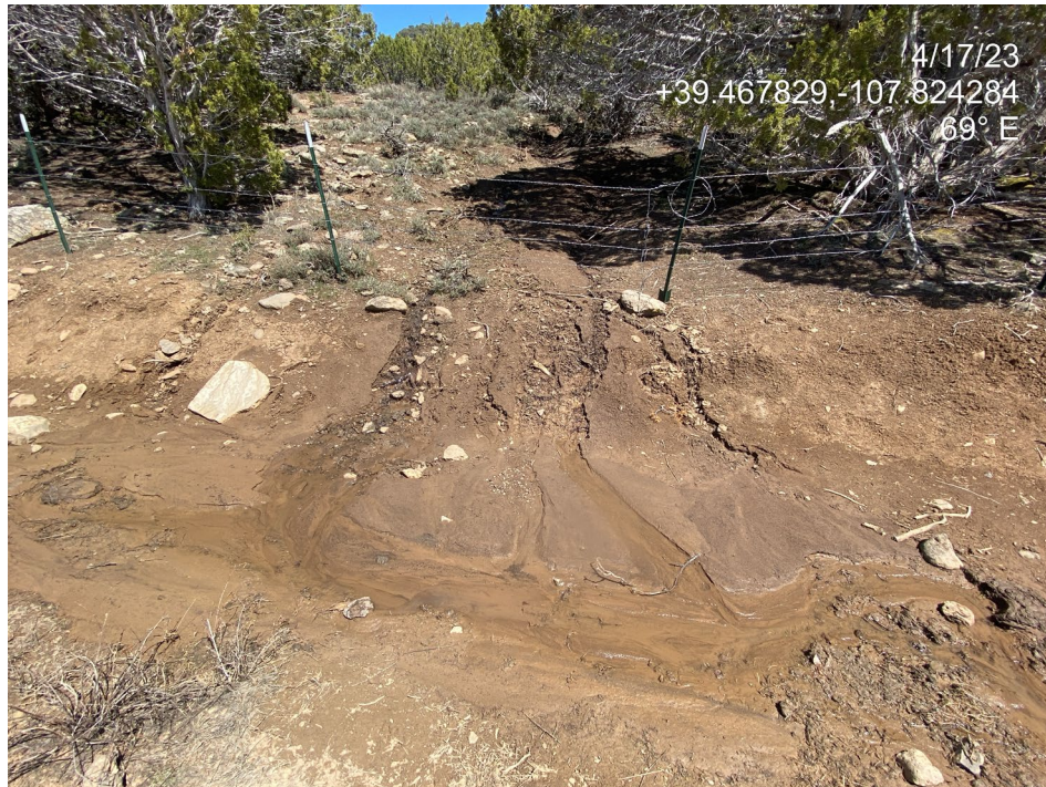
Photo 10. Photos show a small portion of the cut at the northeast of the location which leads into a stormwater ditch is unstabilized.
