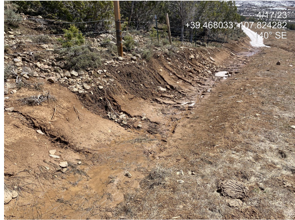
Photo 10. Photos show a small portion of the cut at the northeast of the location which leads into a stormwater ditch is unstabilized.
