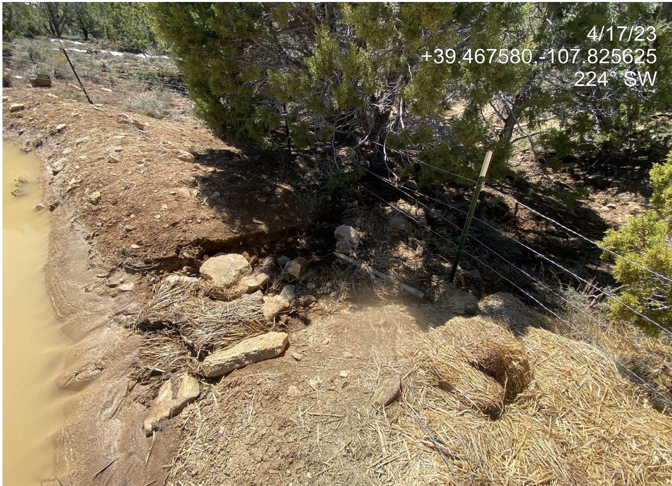
Photo 14. Photos show insufficient sediment trap outlet protections/degraded BMPs.
