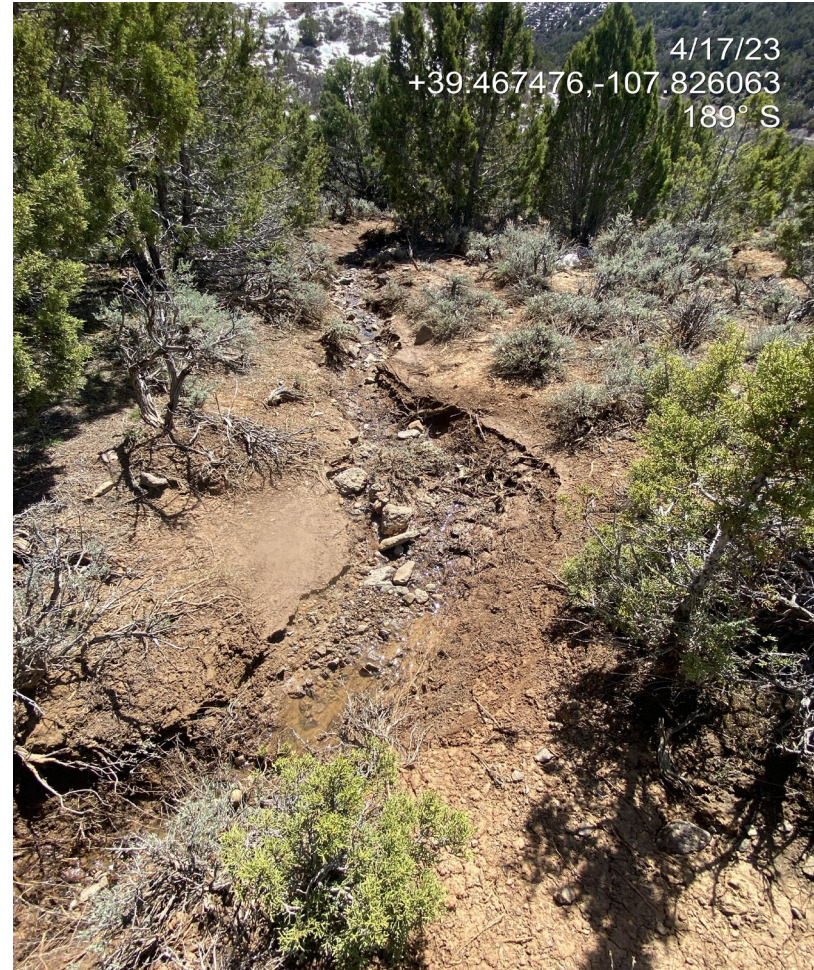
Photo 15. Photos show offsite degradation downslope of the sediment trap outlet pictured in Photo 13.
