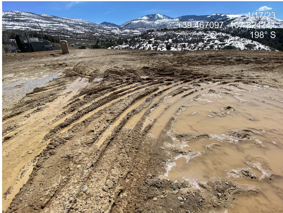
Photo 5. Photos show lack of stabilization of the pad surface.
