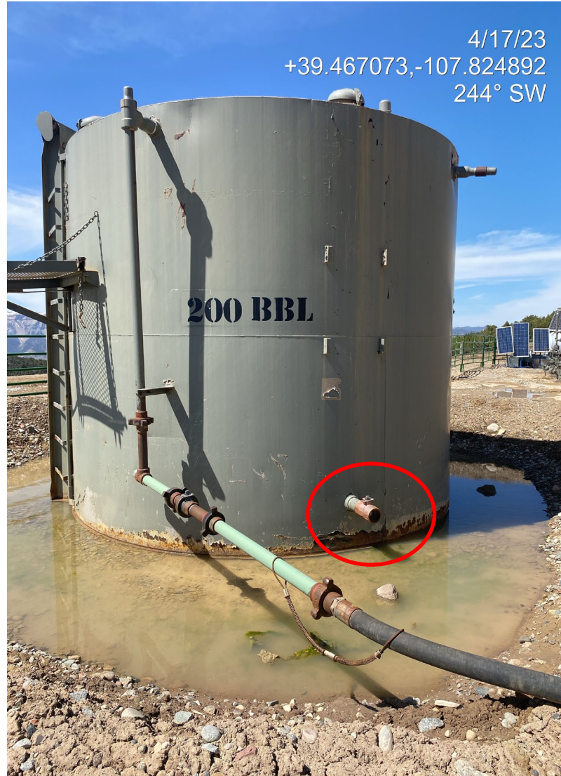
Photo 3. Photo shows a bull plug not installed on a tank drain.
