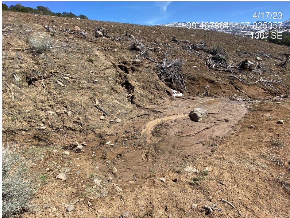
Photo 12. Photos show a sediment trap at the northwest of the location. The interim area above and side of the trap is not stabilized.
