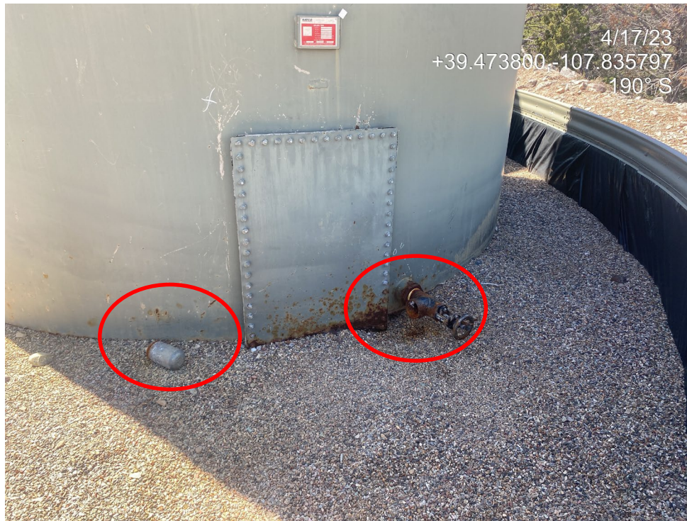
Photo 4. Photos show a bull plug not installed on a tank drain (left) and wildlife protection BMPs in disrepair (right).
