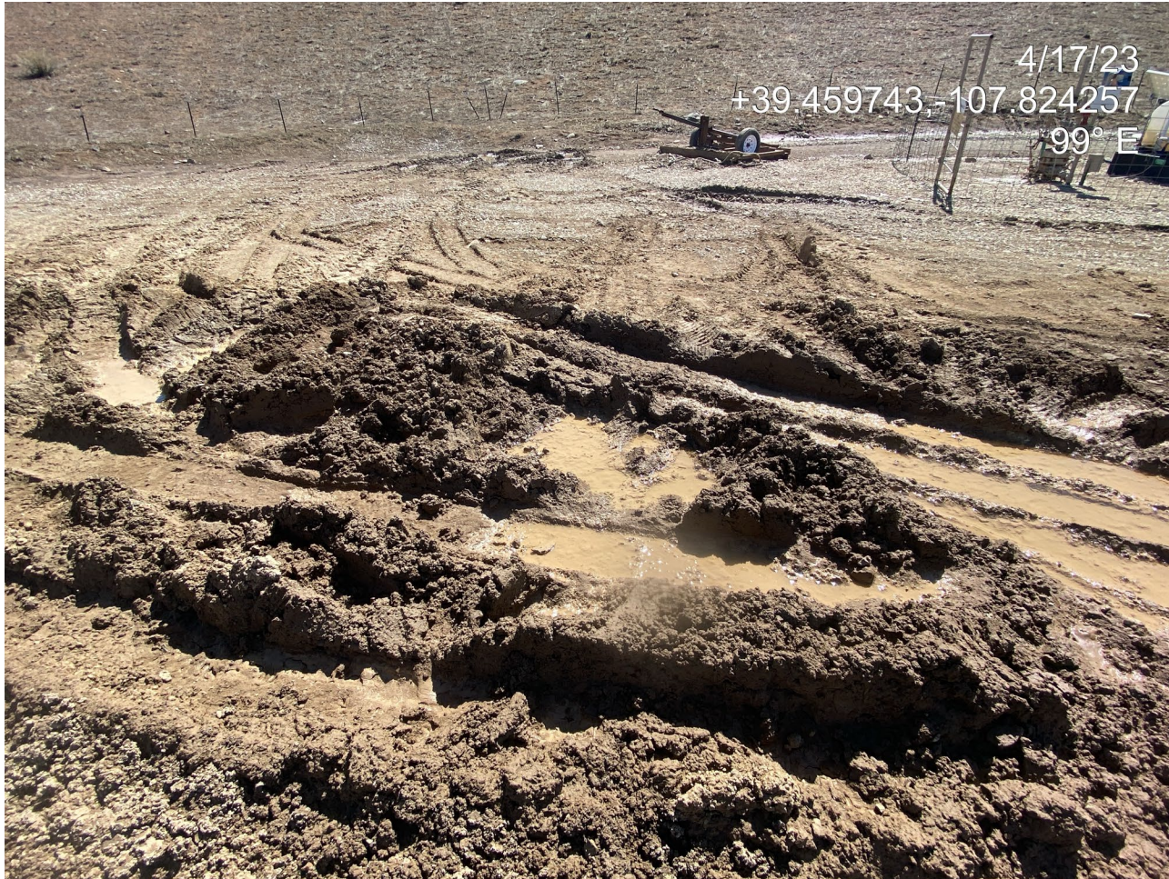
Photo 4. Photo shows lack of stabilization of the pad surface.
