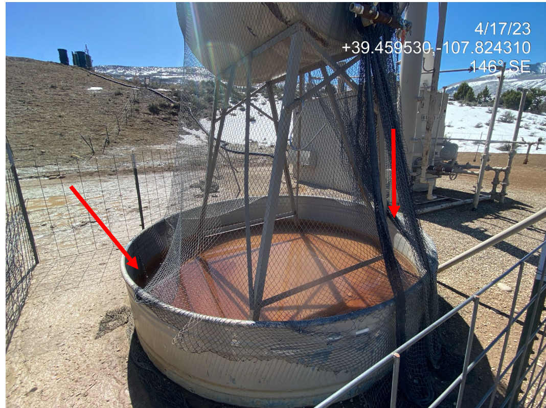
Photo 3. Photo shows wildlife protection netting in disrepair.
