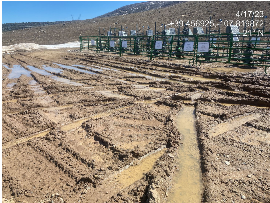
Photo 4. Photos show a lack of stabilization of the working pad (left) and access road (right).
