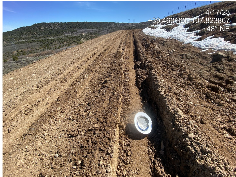
Photo 4. Photos show a lack of stabilization of the working pad (left) and access road (right).
