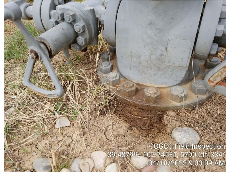
Photo #18 – Localized accumulation of oily waste observed at C35 Kell 35-3 wellhead.
