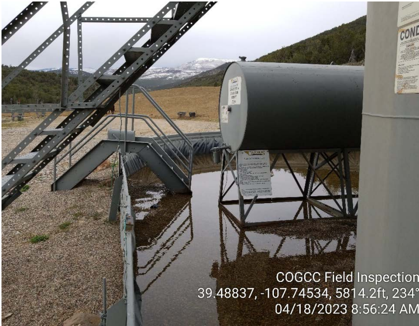
Photo #11 – South half of tank battery secondary containment contained hydrocarbon-impacted fluids on inspection date.
