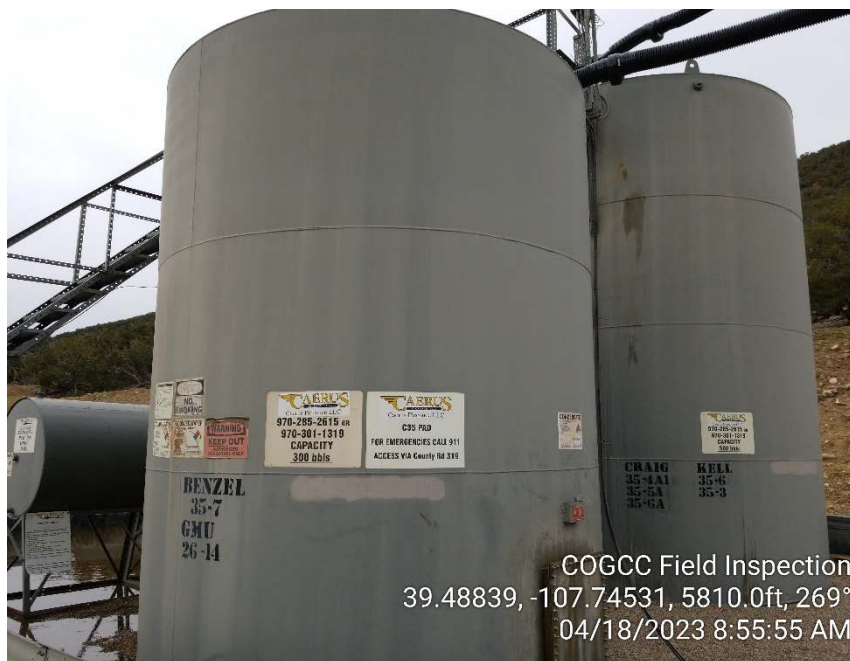
Photo #9 – Tank battery consists of one 300 bbl steel AST and one 500 bbl steel AST, both labeled to contain Produced Water and Condensate, and one 24 bbl methanol tank inside of a lined metal berm.
