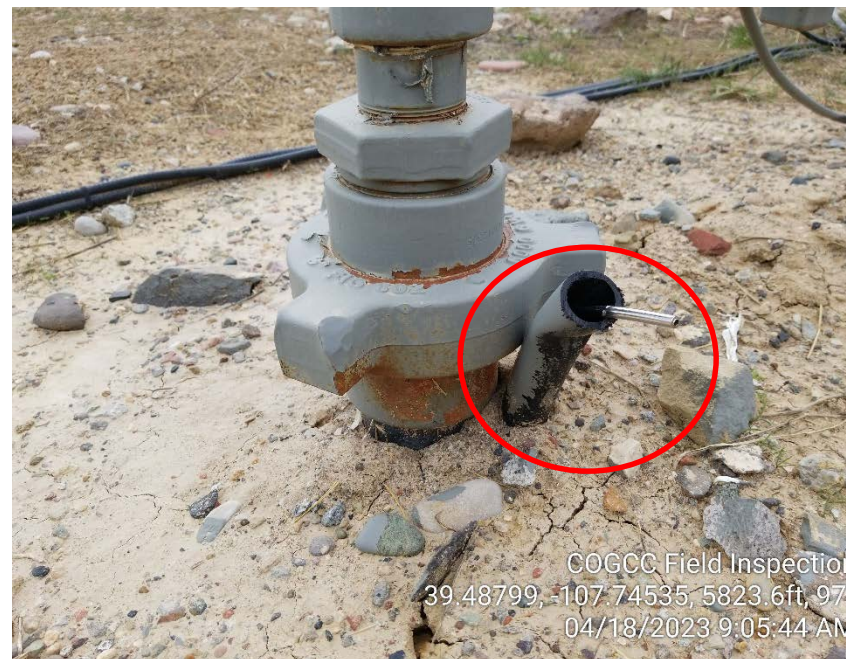
Photo #20 – Multiple wellheads (GMU 35-4A1, Craig 35-6A, and Craig 35-5A) have associated flowline risers configured with an uncapped 1/4" process pipe.
