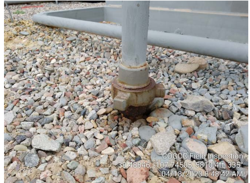
Photo #6 – Staining and discoloration observed at hammer union on Kell 35-3 Separator.
