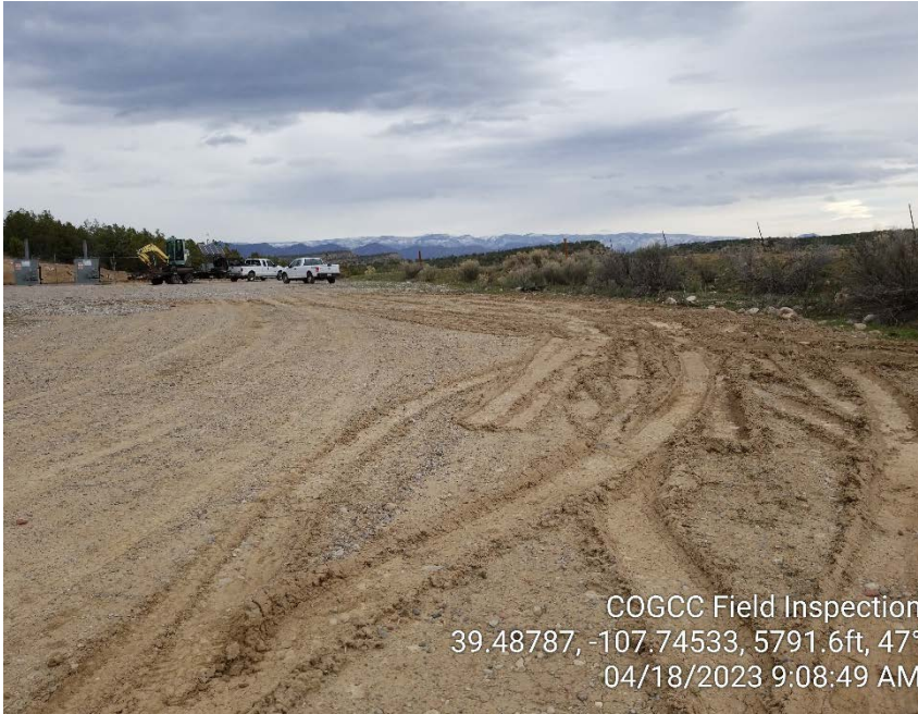
Photo #23 – Rutted area along east side of pad.
