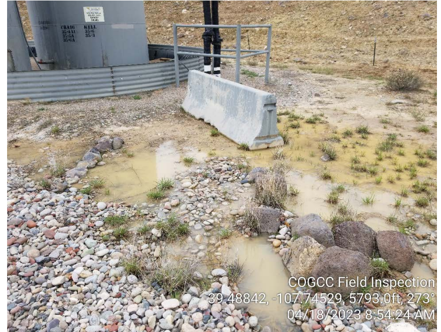
Photo #8 - Stormwater pooling on north side of tank battery.
