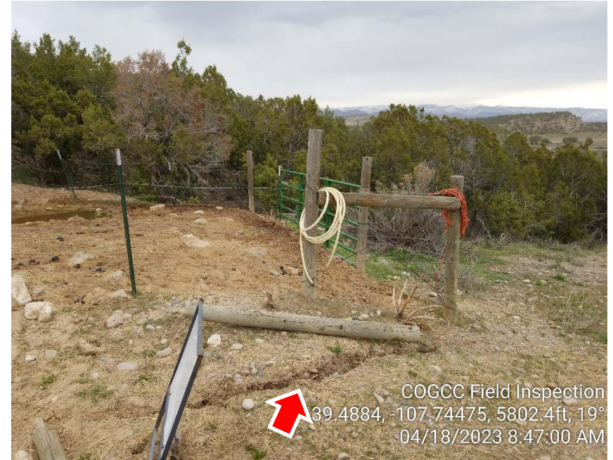
Photo #2 – Additional debris (fence post and rope) at entrance to pad. Note erosion rill located between sign and fence (red arrow).
