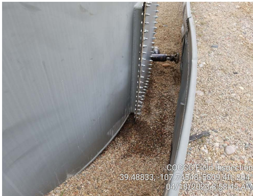
Photo #13 - Localized accumulation of oily waste near manhole cover and bullplug attached to 500 bbl steel AST has the potential to impact stormwater accumulations.
