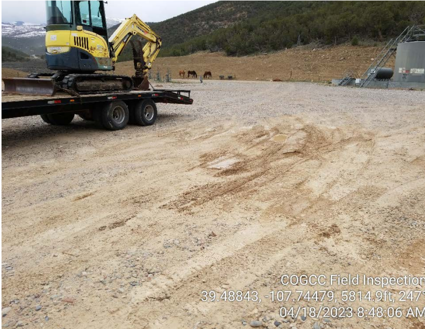
Photo #5 – Ruts, erosion, and sediment transport were observed throughout the pad surface on inspection date.
