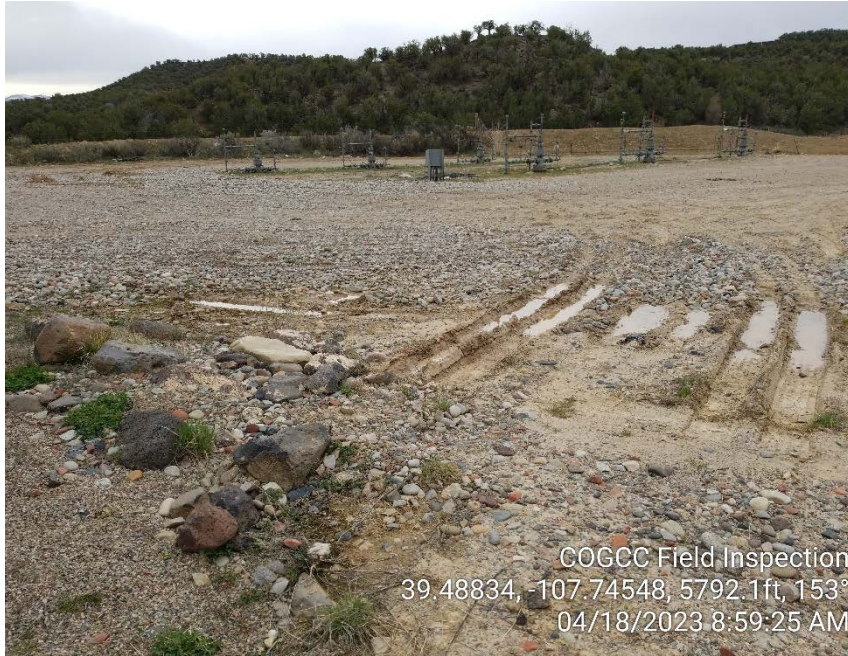
Photo #15 – Ruts and stormwater accumulation on pad.
