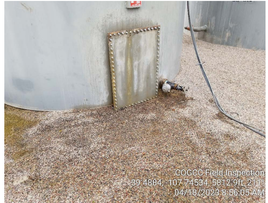
Photo #12 - Localized accumulation of oily waste near manhole cover and bullplug attached to 300 bbl steel AST has the potential to impact stormwater accumulations.
