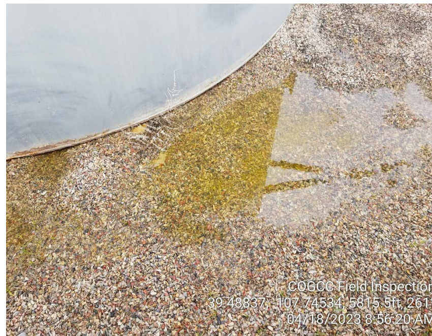
Photo #10 – Tank battery secondary containment contained unknown fluids on inspection date. Discoloration of fluids in close proximity to 300 bbl steel AST indicate potential hydrocarbon impacts.
