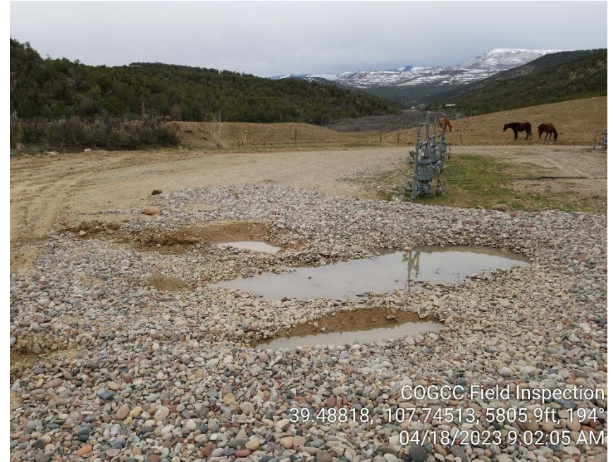
Photo #16 – Stormwater accumulation and ruts on pad.
