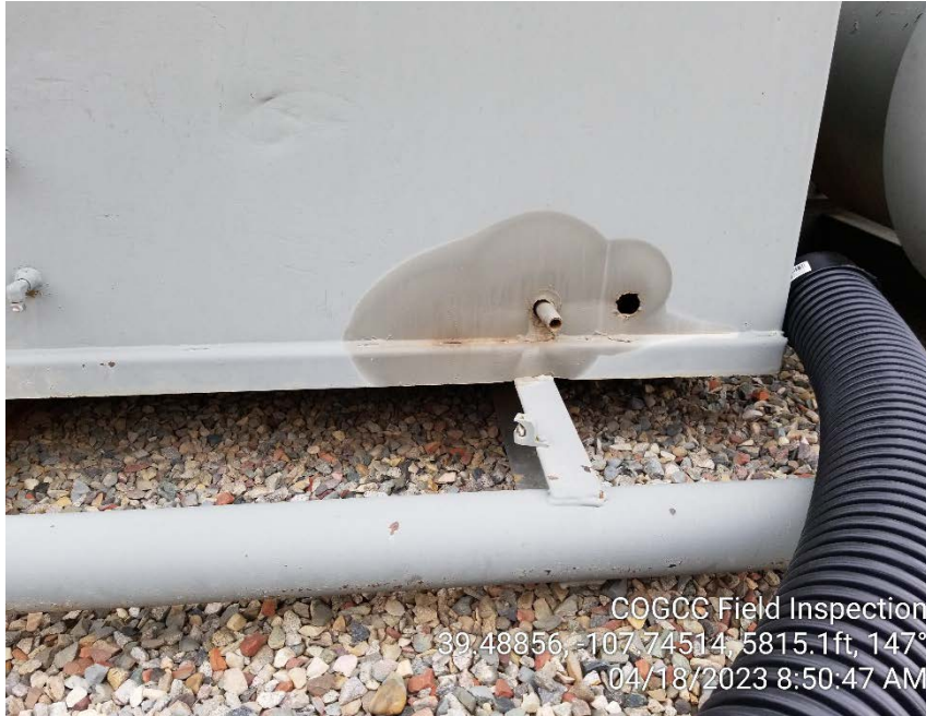
Photo #7 – Fluid staining observed on west side of vertical separator for Craig 35-5A C35 well.
