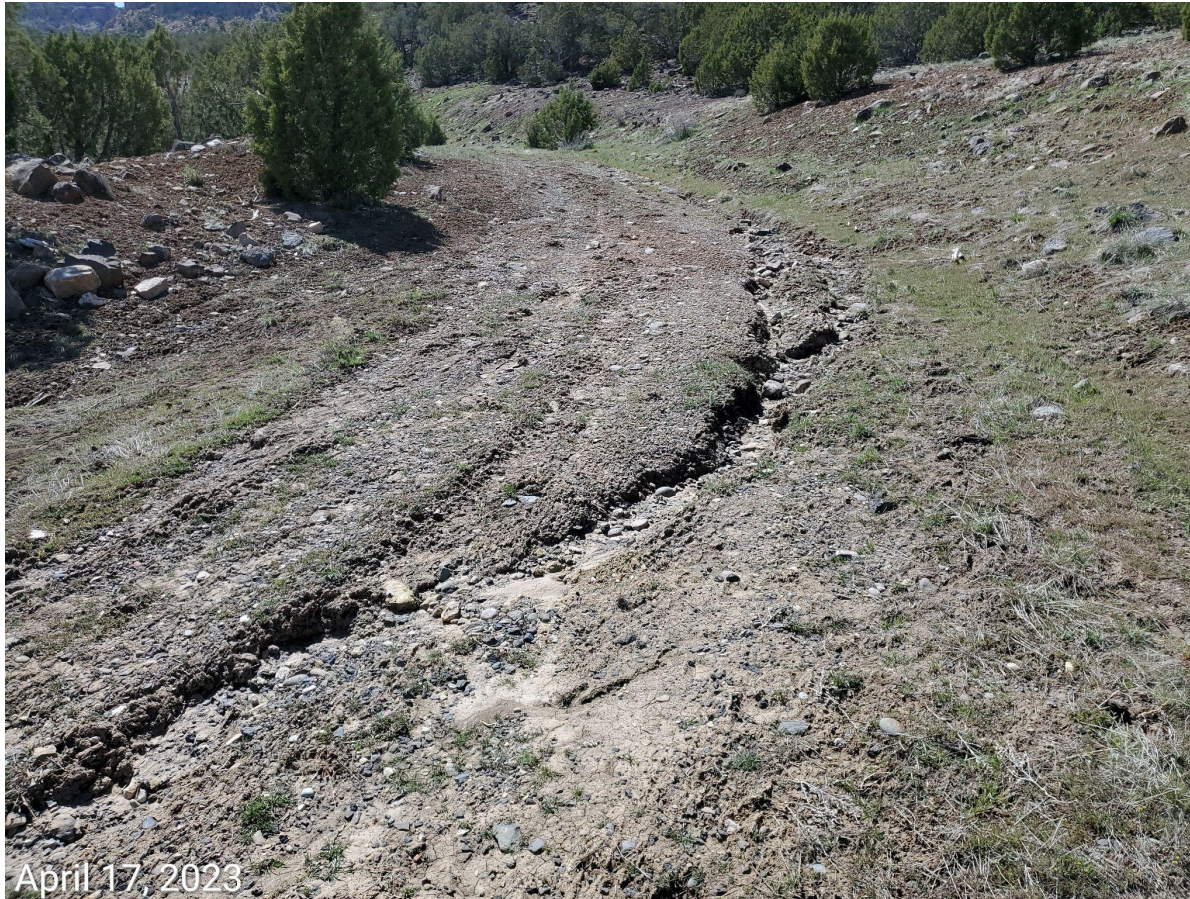
Photo 16: Erosion degradation at the access road.
