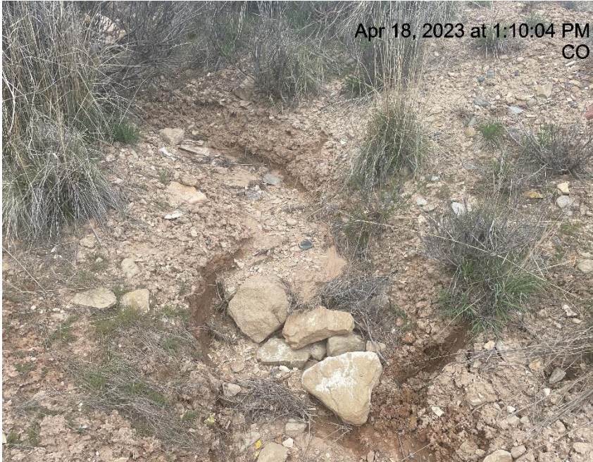
Photo # 5670 Check dam needs maintenance (SW corner of lower pad that wellheads are located on)
