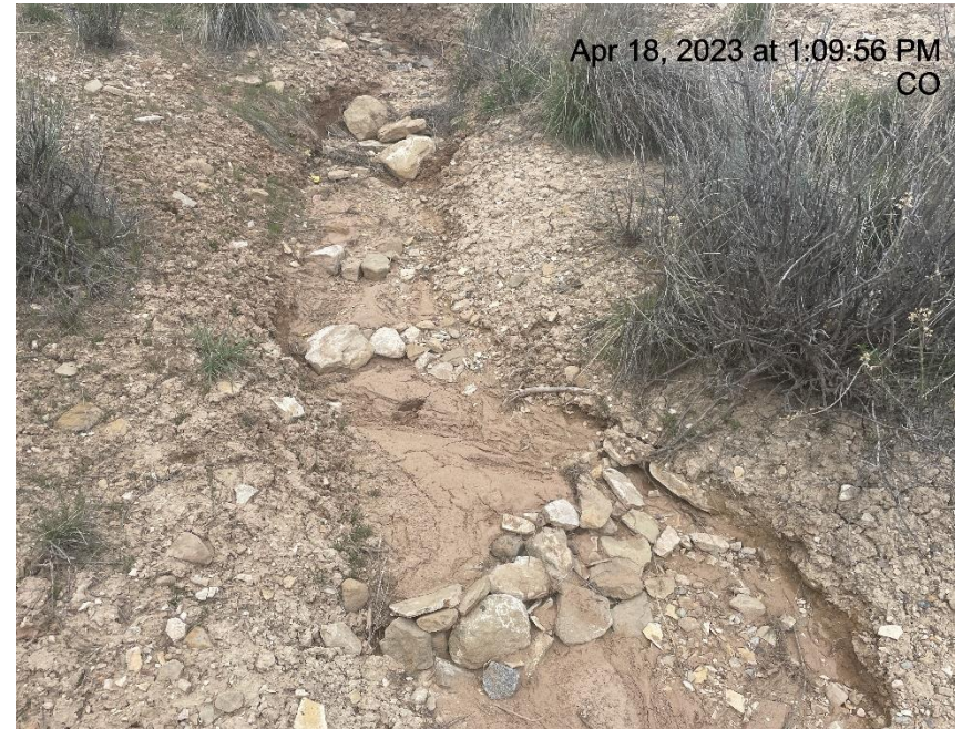
Photo # 5669 Check dams need maintenance (SW corner of lower pad that wellheads are located on)
