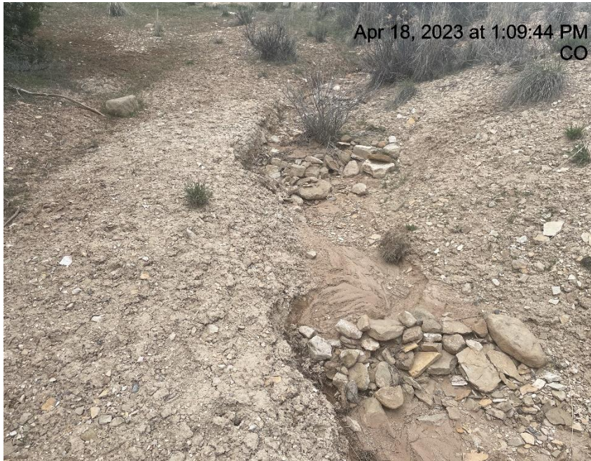
Photo # 5668 Check dams need maintenance (SW corner of lower pad that wellheads are located on)
