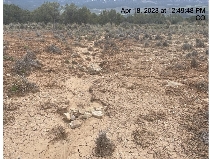
Photo # 5633 Check dams need maintenance (SW area of pad)
