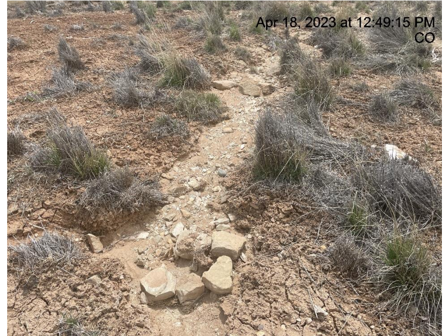
Photo # 5631 Check dams need maintenance (SW area of pad)
