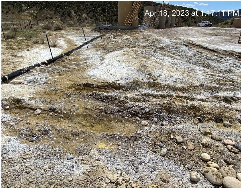
Lack of stabilization and sediment migration
