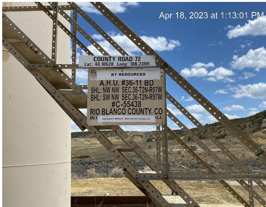
API Number missing from tank battery sign
