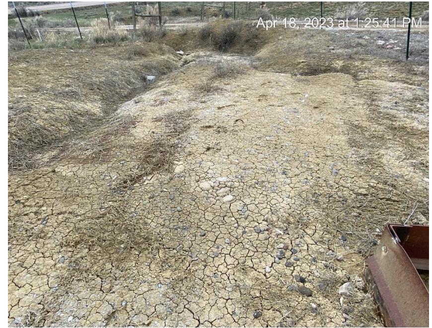
Erosion and sediment migration
