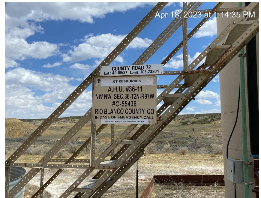
API Number missing from tank battery sign
