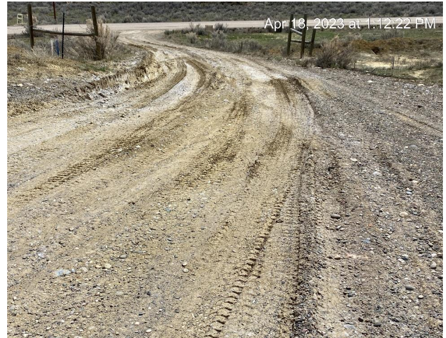
Access road to location
