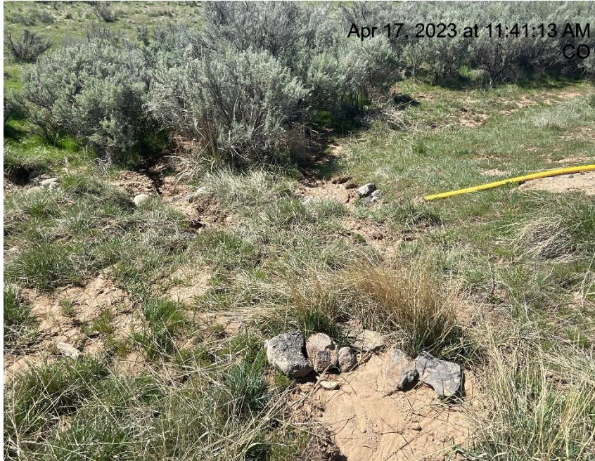
Photo # 5467 Erosion & transport of sediment off location/insufficient BMP's (SE area of location, near entrance to location)
